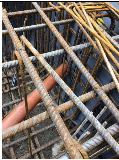
Internal section of pipe within pile cap
