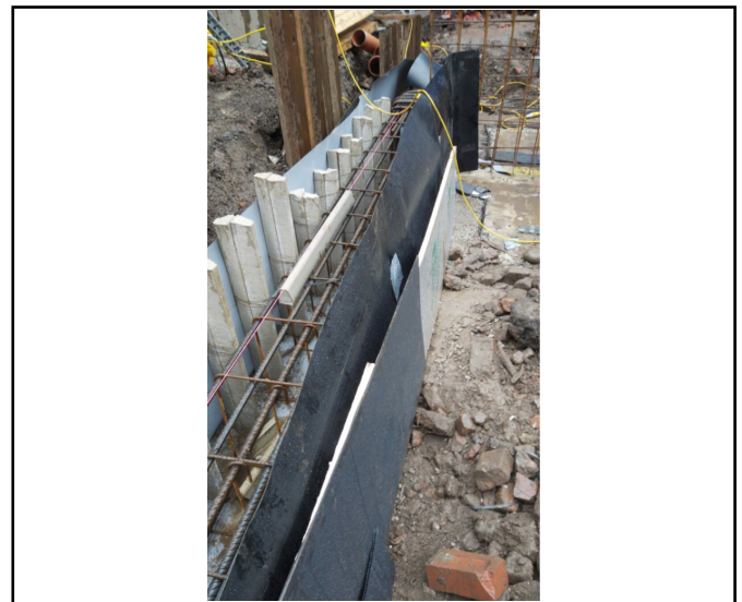
Ring beam showing wrapped membrane
