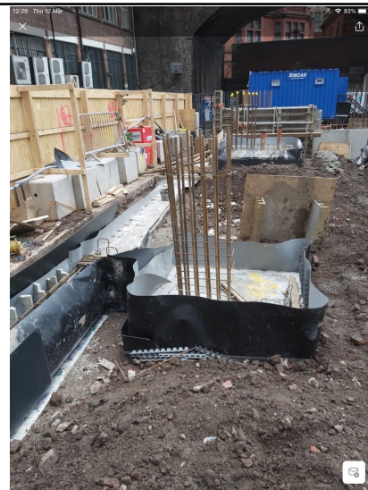
Pile cap and ring beam, both have
