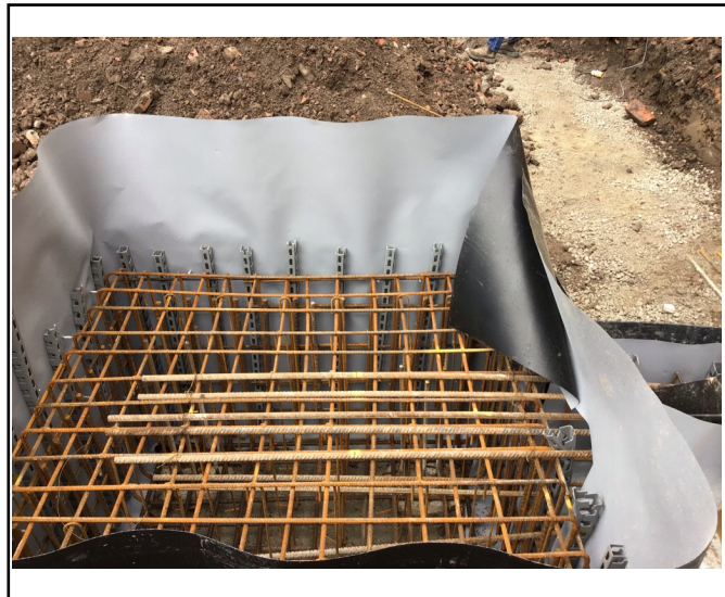
Pile cap with Visqueen Geoseal
