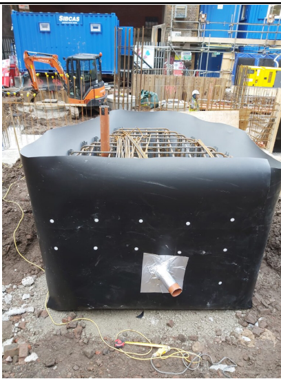
External pipe from above right photo
