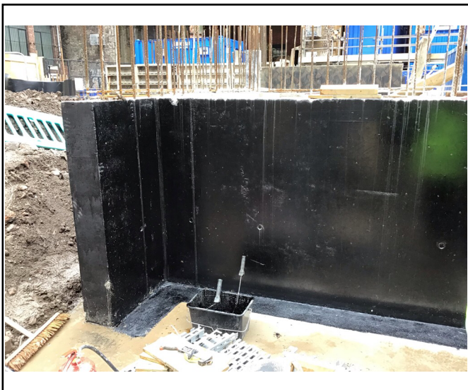
Primed wall with bucket of primer
