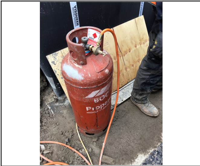
Gas used to prime bitumen
