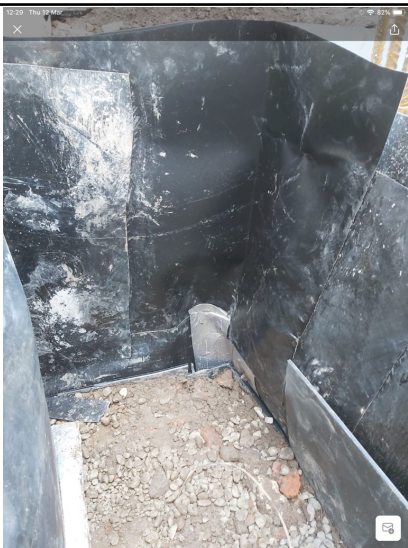
Exterior corner detail of Visqueen
