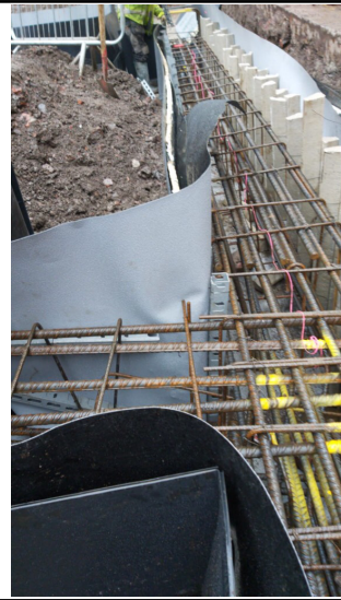
Overview of ring beam with visqueen
