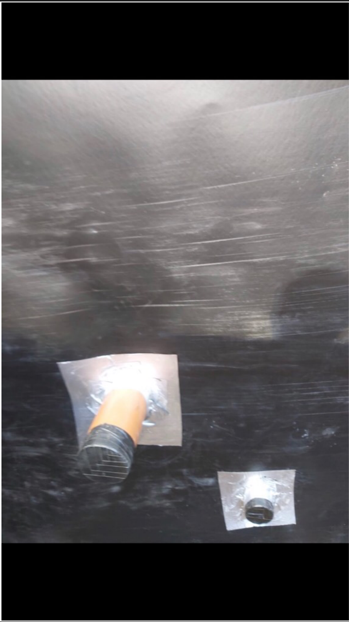
Above photo) external pipe work sealed with GR SAM
