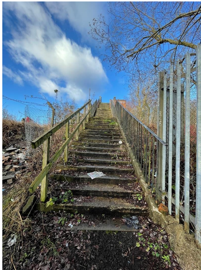
Photograph 5: Stairway at southern extent of Lowry Footbridge
