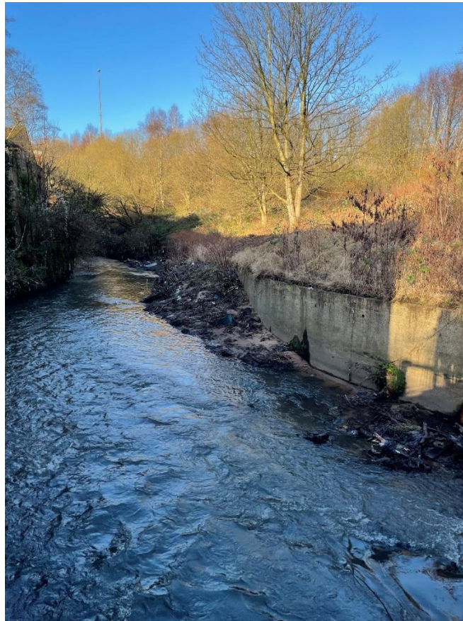
Photograph 6: Concrete riverine walls along northern bank of the River Irk, camera facing northwest from Catherine's Wood footbridge
