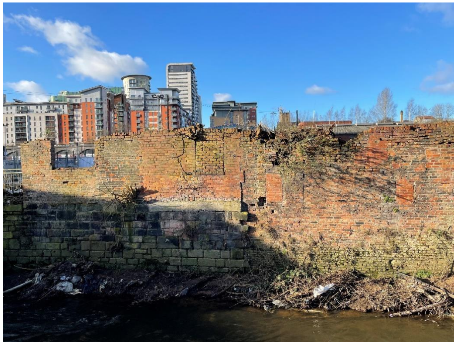
Photograph 8: View facing north of different phases of stone and brick riverine walls in southwest corner of site, immediately upstream from Union Bridge
