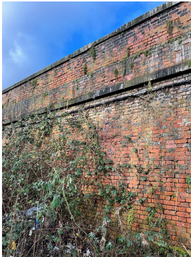
Photograph 9: Industrial red brick retaining wall, camera facing north
