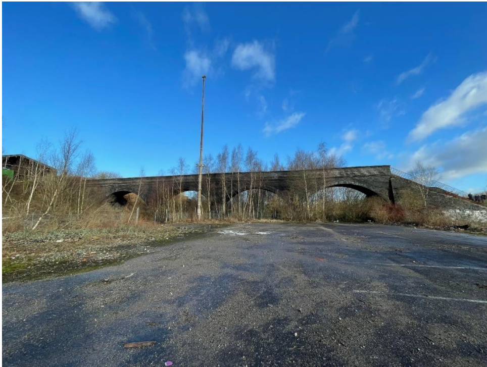
Photograph 3: View of Lowry Footbridge, camera facing northeast
