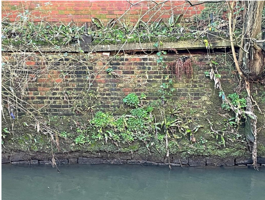
Photograph 7: Historic red brick riverine and stone walls along southern bank of the River Irk
