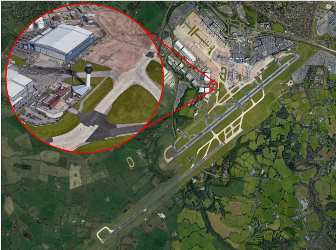
Figure 8 ATC Tower location
