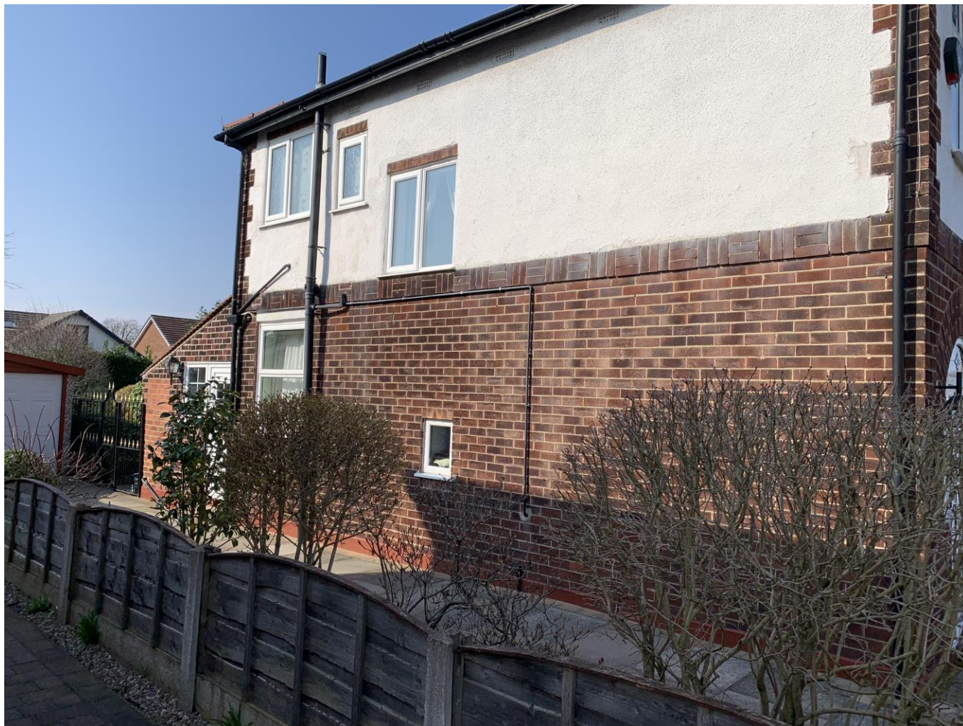
Photograph 2 Side Elevation of no.9 Sandilands Road, (Source: Officers Photographs taken on 08.03.2022)
