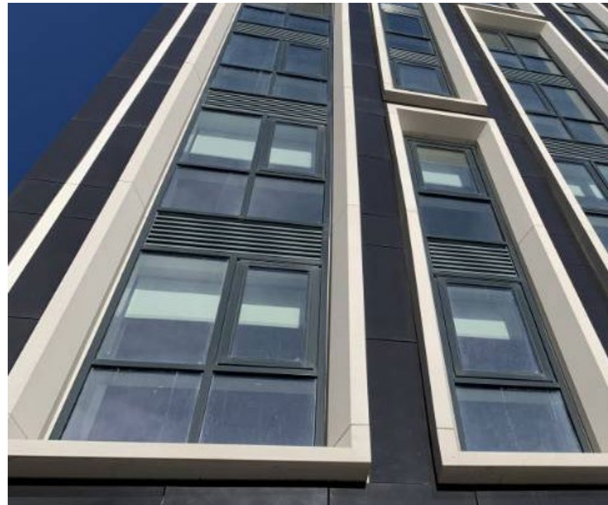
21 STRAND STREET - TEXTURED PANEL
