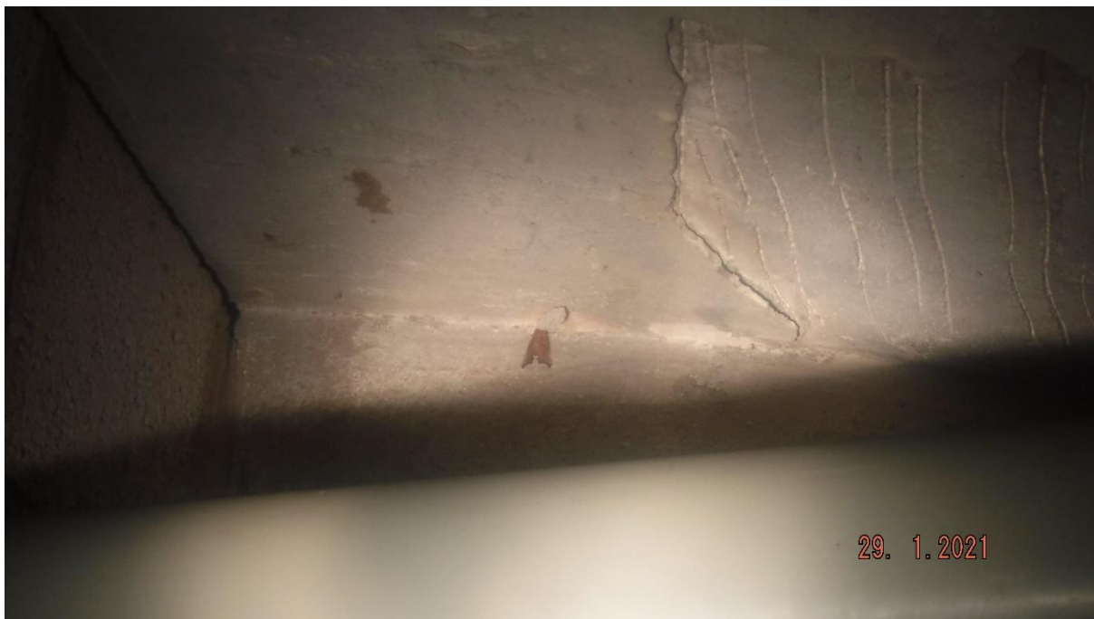
Photo 8. Herald moth identified within the basement in January 2021.
