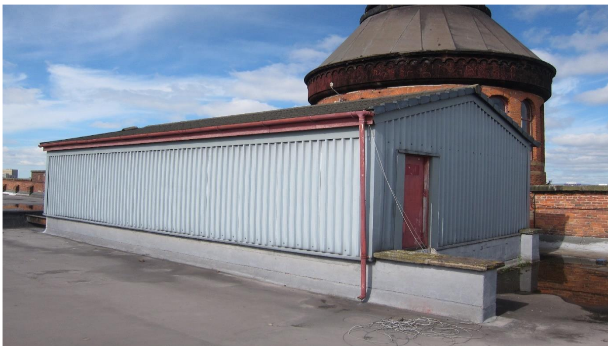
Photo 3. Motor building associated with lift shaft on top of the roof of Victoria Mill.
