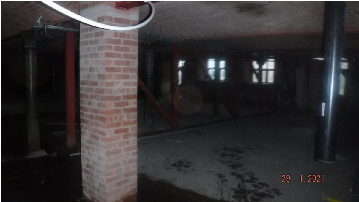
Photo 7. Looking south-west towards the courtyard from the largest room of the basement.
