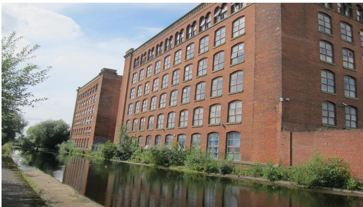
Photo 2. Rear (south-eastern) aspect of Victoria Mill with Rochdale canal also visible.
