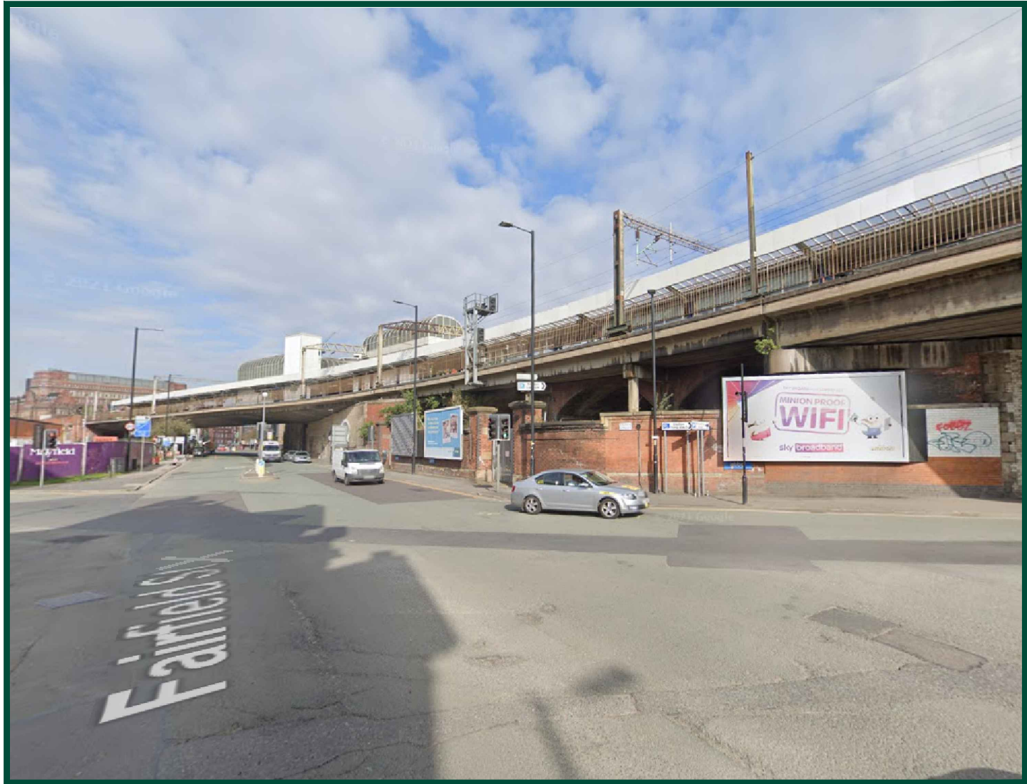
EXISTING SITE VIEW
