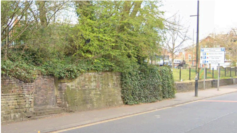
Remnants of access from Stockport Road within retaining wall
