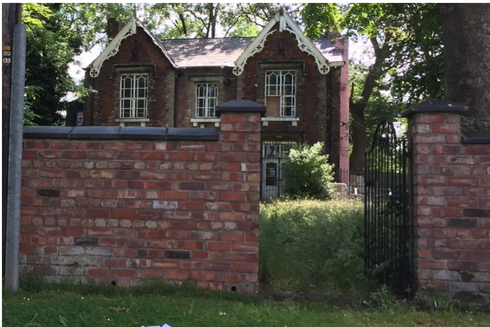
Boundary wall & pedestrian gate facing open grassed area.
