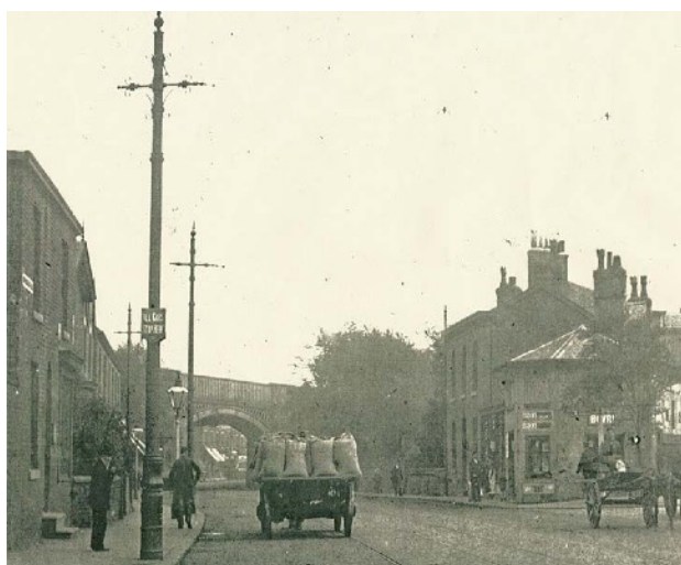
View of intersection between Slade Lane & Stockport Road
