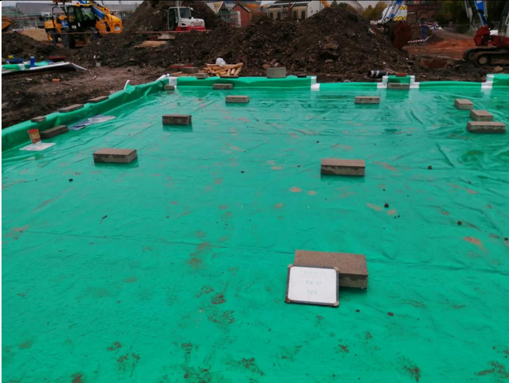
Photograph 5: Validation of Gas Membrane Installation
