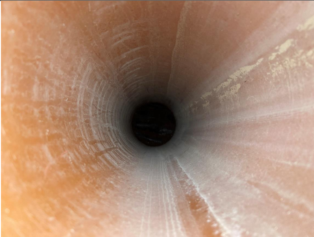
Photograph 3: Validation of Geotextile Membrane
