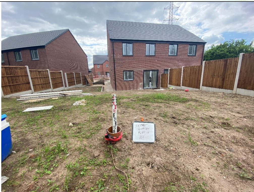
Photograph 2: Validation of Garden Capping Thickness (Plot 52, not 51)
