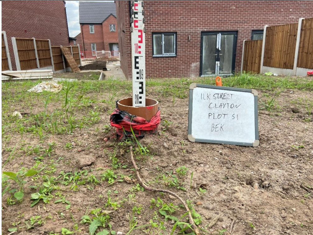
Photograph 1: Validation of Garden Capping Thickness (Plot 52, not 51)
