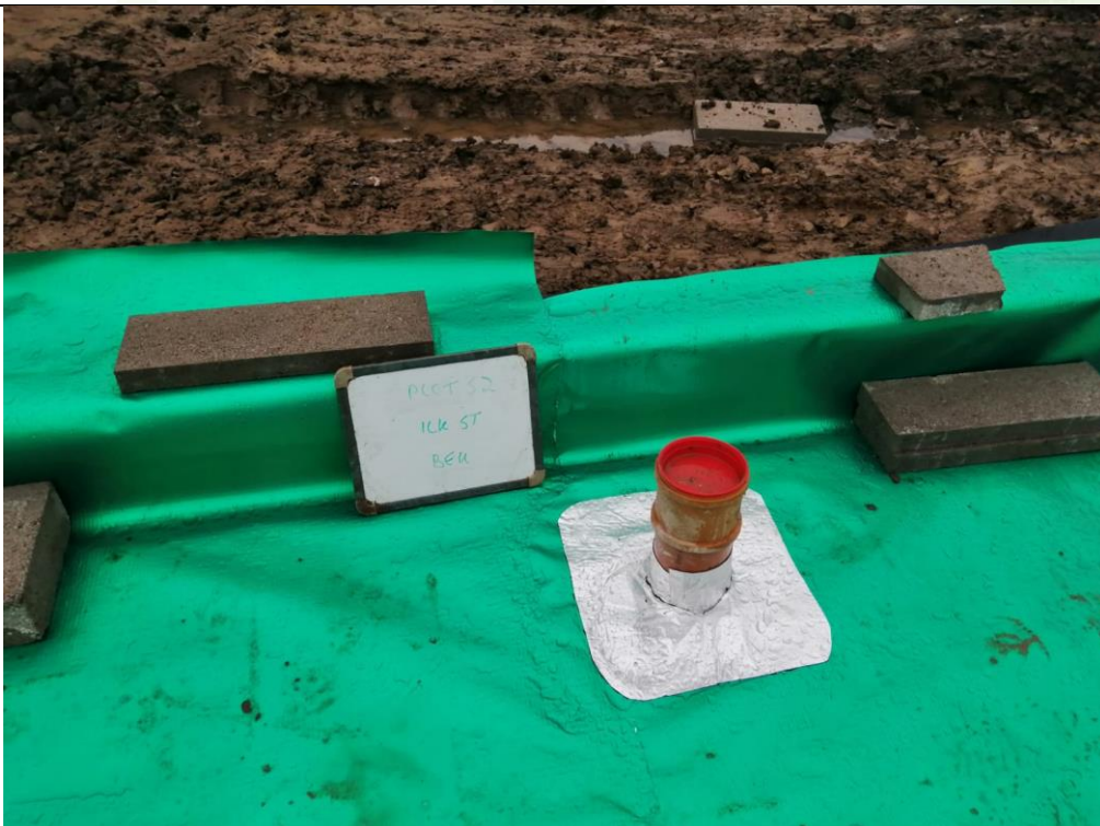
Photograph 6: Validation of Gas Membrane Installation
