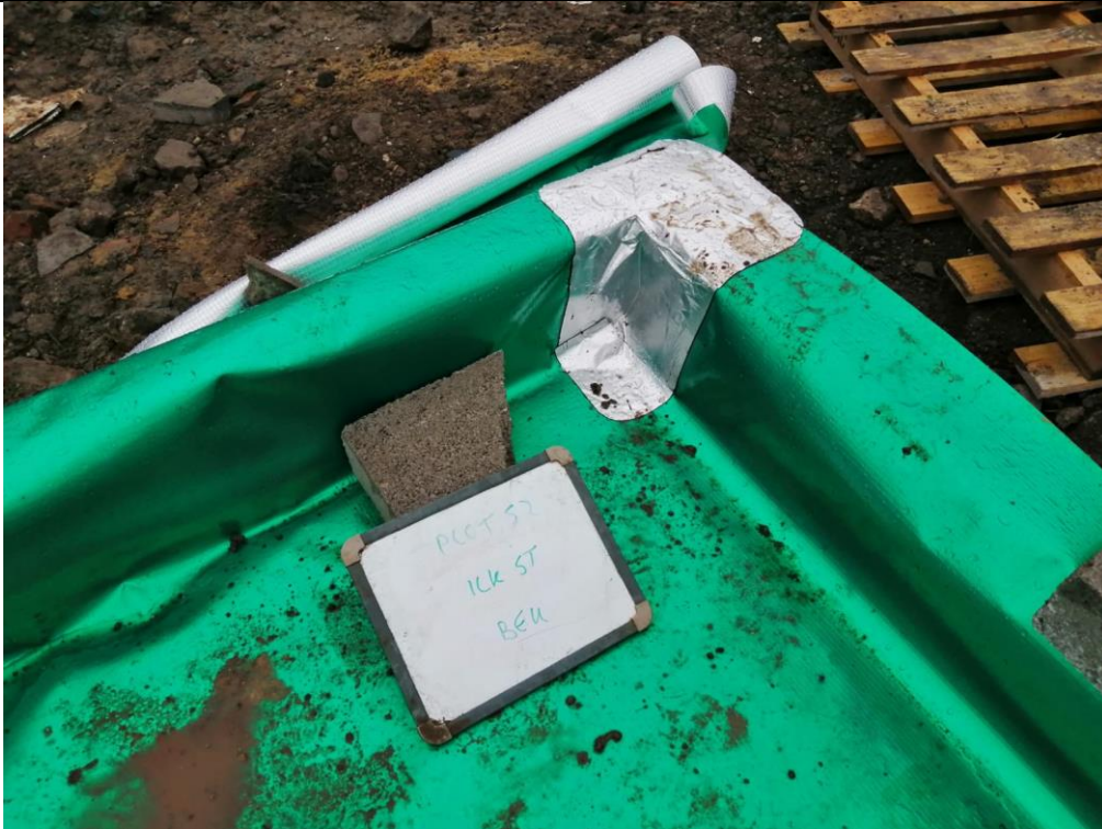
Photograph 7: Validation of Gas Membrane Installation
