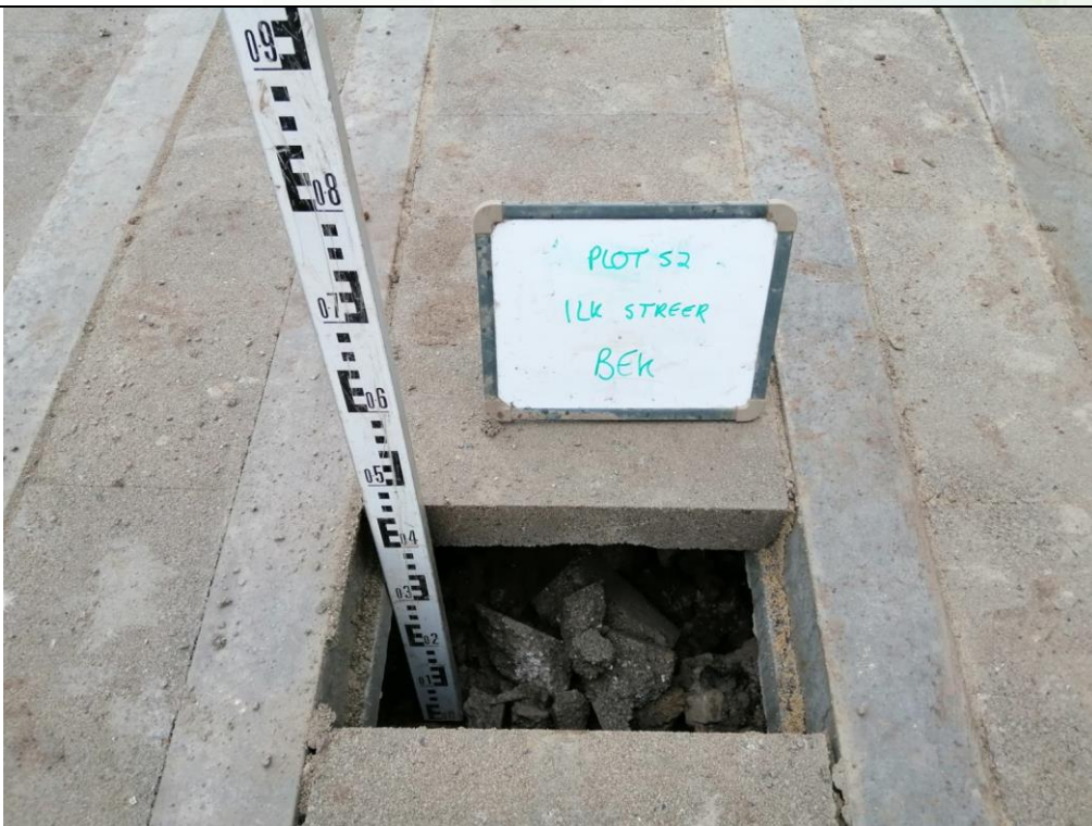
Photograph 4: Validation of Sub-Floor Void Space (min 150 mm)
