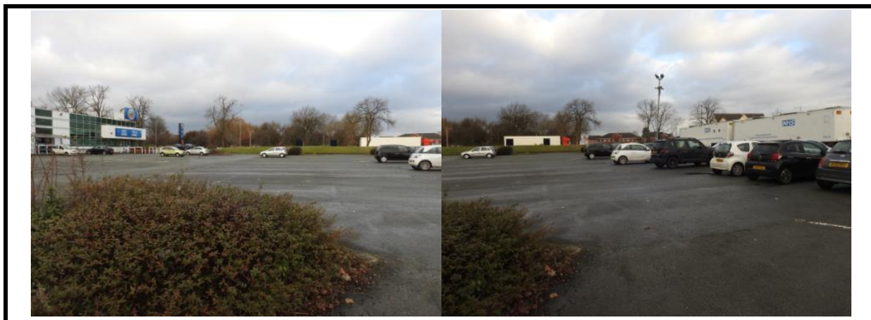
Car park are for both units.
