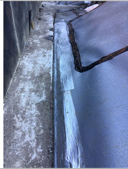
Link at perimeter sealed
