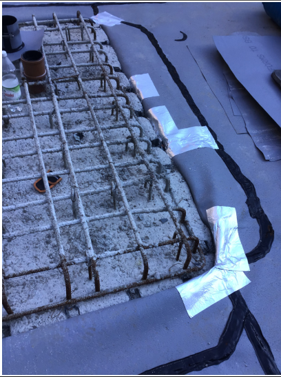
Corners to piles caps now sealed
