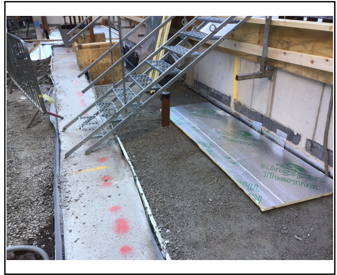
Membrane to connect ring beam
