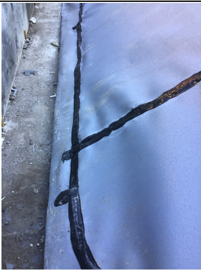
Extrusion welds on the slope
