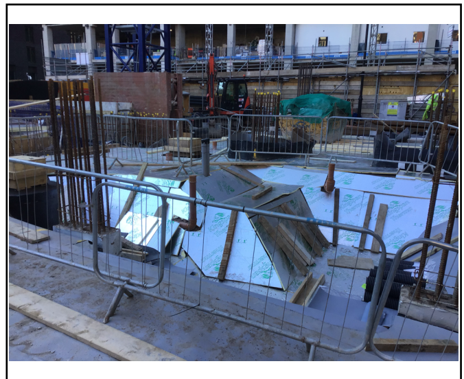
Overview of Gridline 5-7 being
