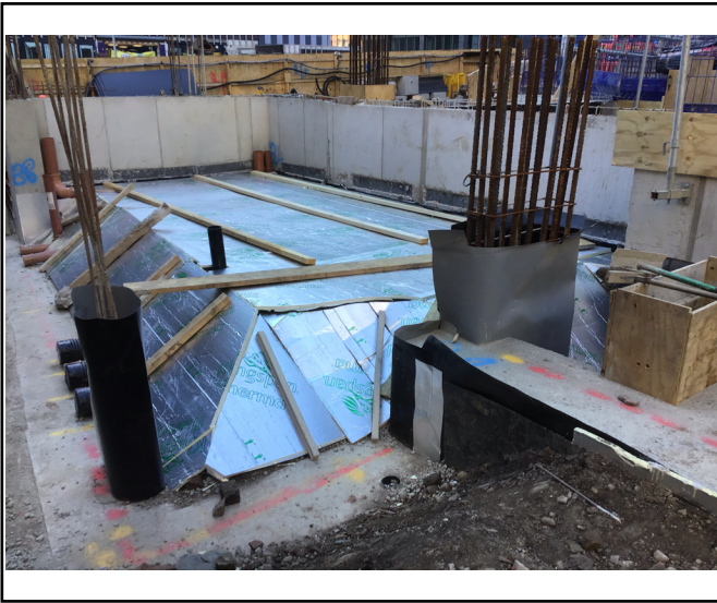
Next section to install in insulation
