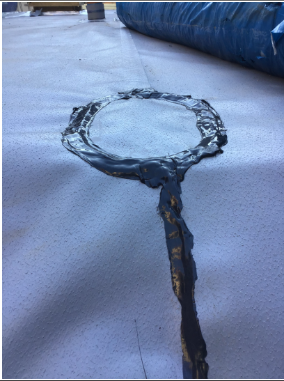
Extrusion welds
