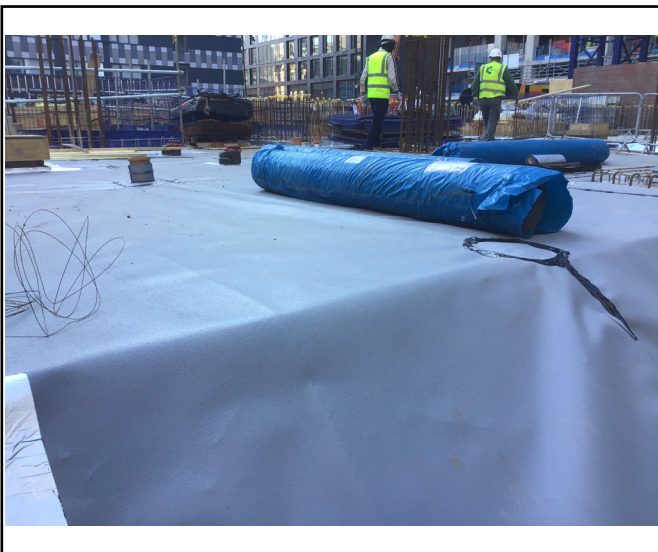
Overview of verified section
