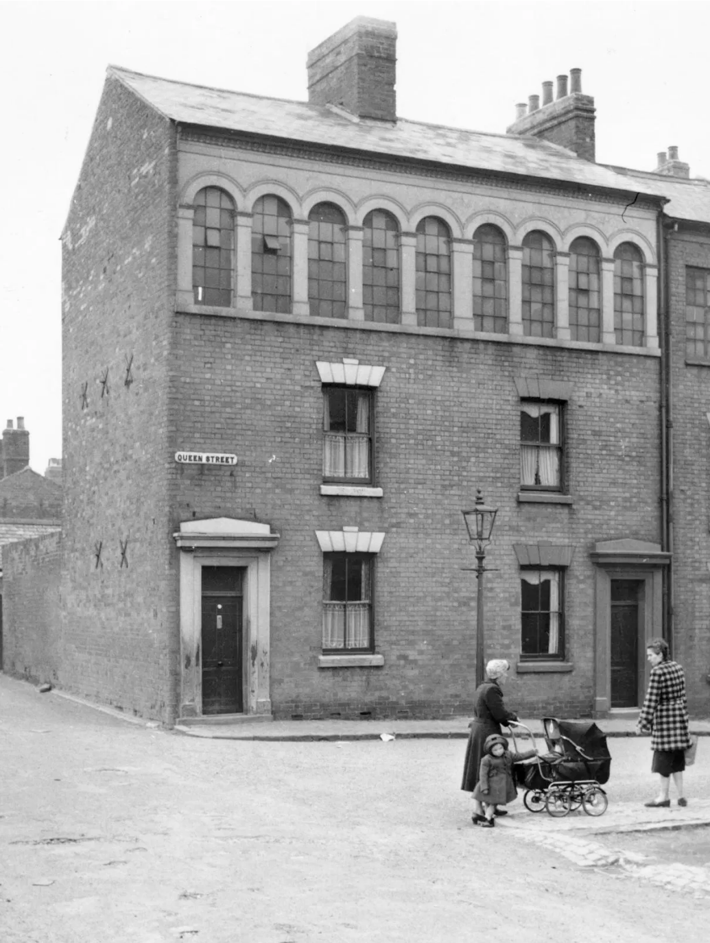
Northern ‘Top-shops’, Reference Historic England. Referencing Manchesters industrial heritage in textile manufacture.
