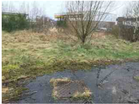
Photograph 4 (P4) Public sewer in the north of the site.
