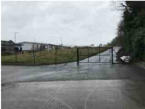
Photograph 1 (P1) Gated access to the site through a driveway off Bury New Road.
