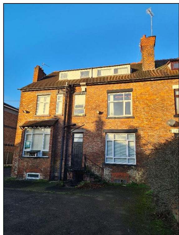
Figure 3: Rear elevation of the subject property.
