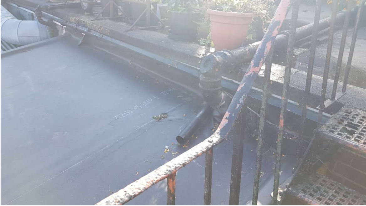
View looking at junction of roof of extension to roof terrace of apartments above
