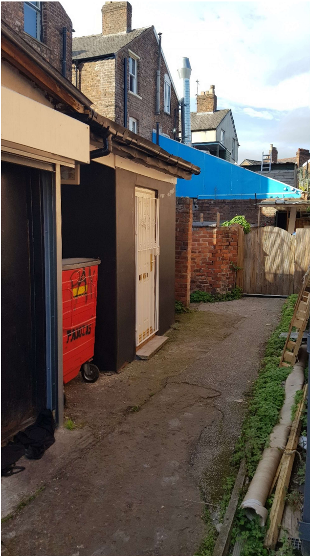
North East elevation of extension with refuse storage area to the left.
