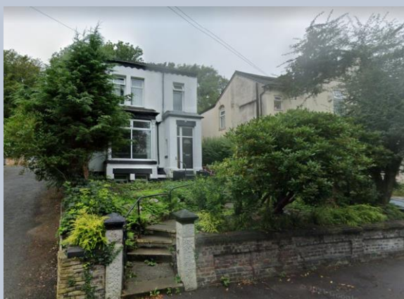
Figure 1: 9A Cleveland Road
