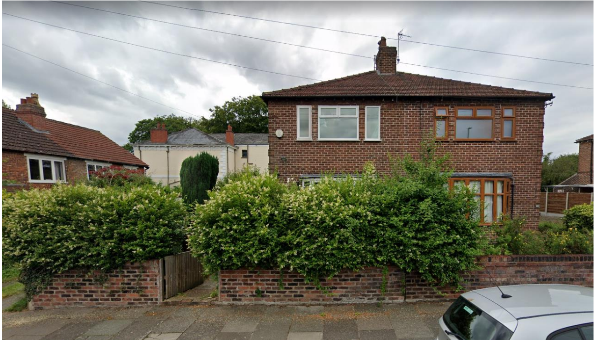
Fig 1. Front Elevation (Google Maps, Street View data, 2022)
