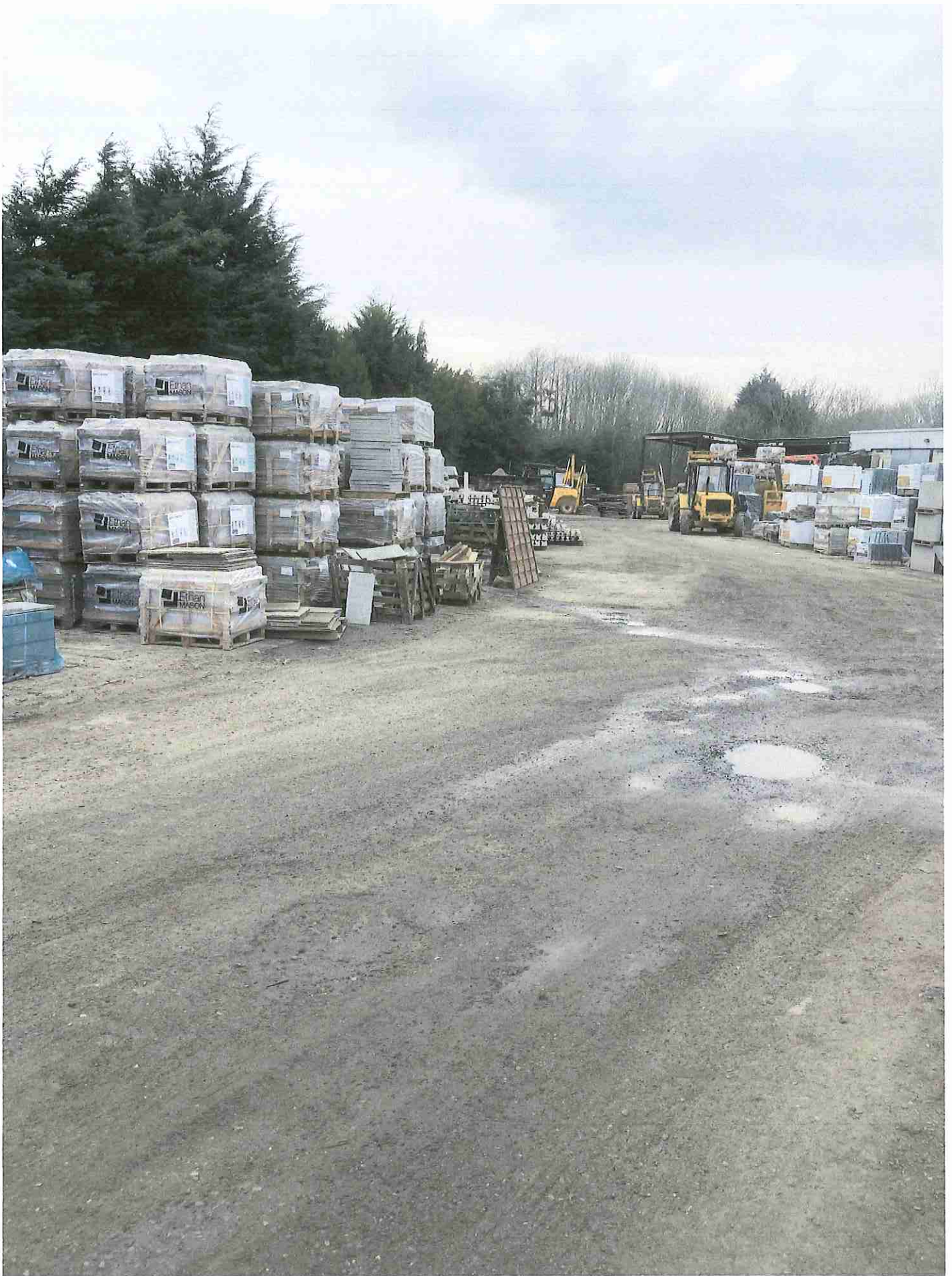
VIEW FROM SITE ENTRANCE
