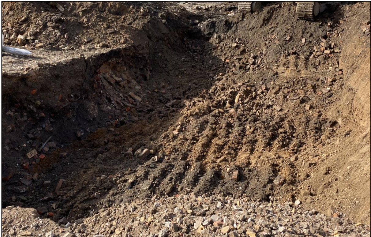
Plate 5: Natural gravel below mixed rubble levelling material, southeast side of the area, looking southeast
