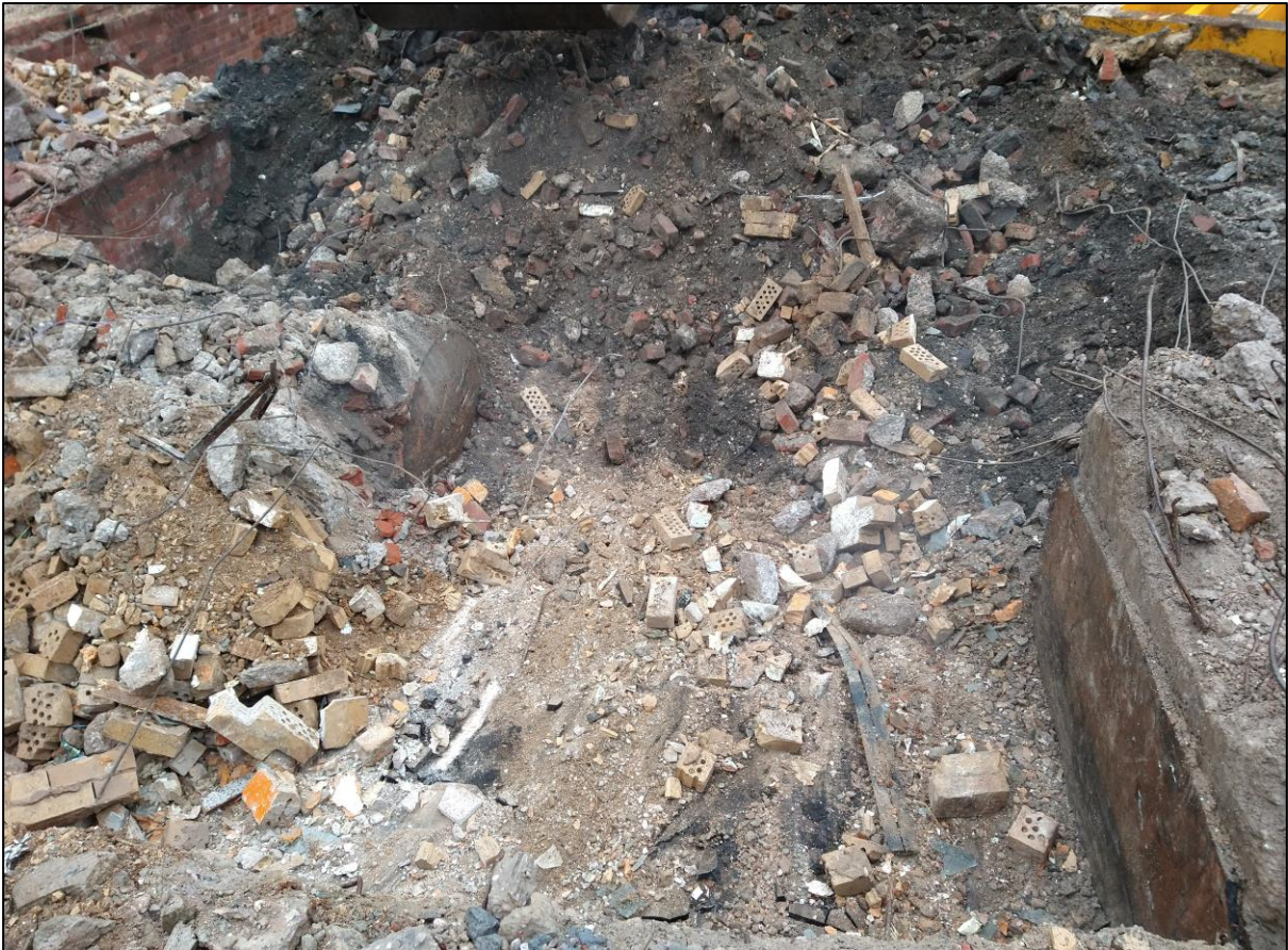
Plate 3: Central basement, note fuel tank at centre left, looking northeast
