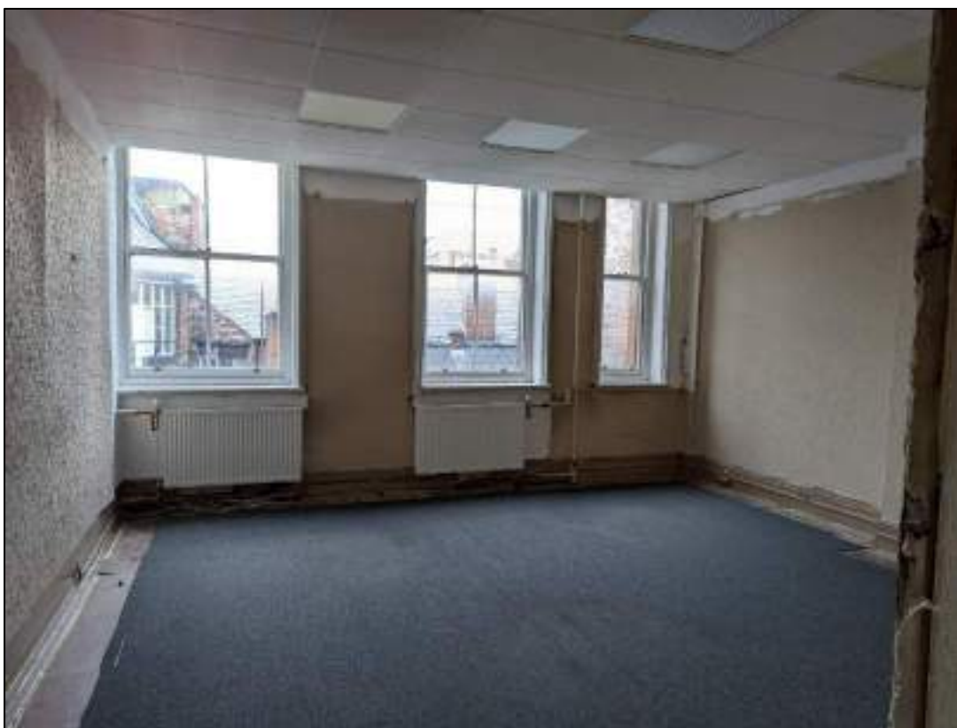
Plate 77: Stripped office space
