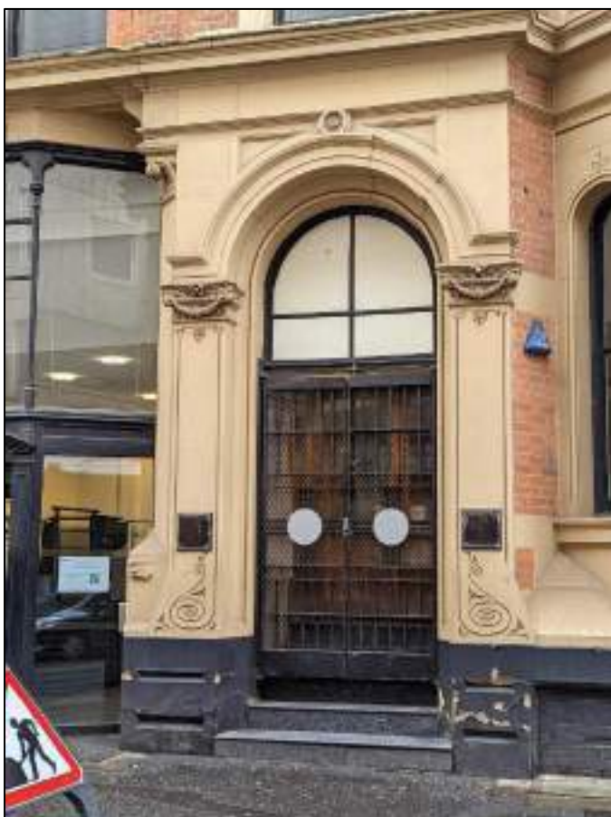
Plate 8: Original hotel entrance in bay 7
