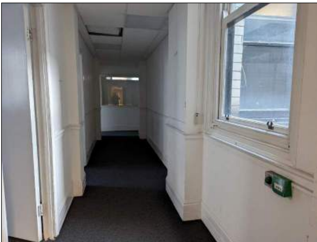
Plate 67: Second floor corridor
