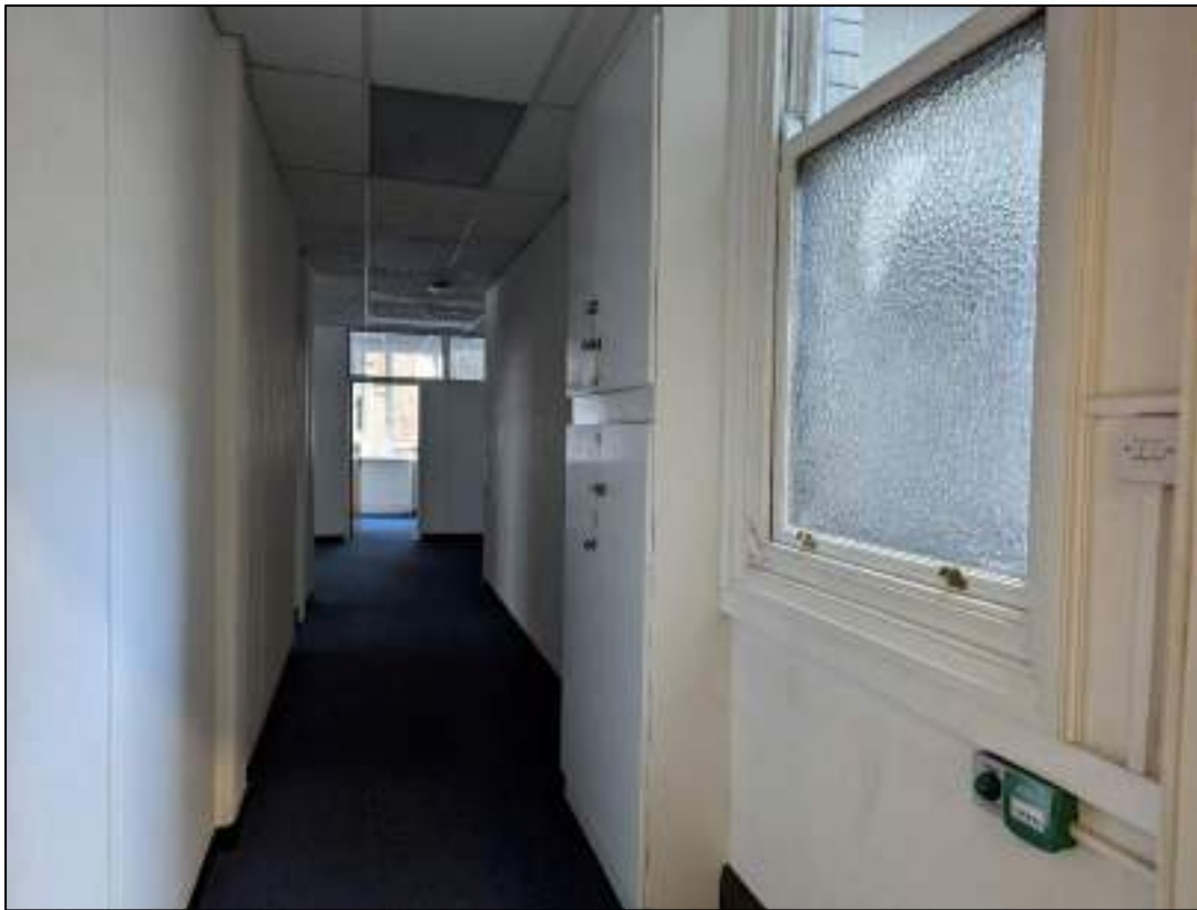
Plate 50: First floor corridor
