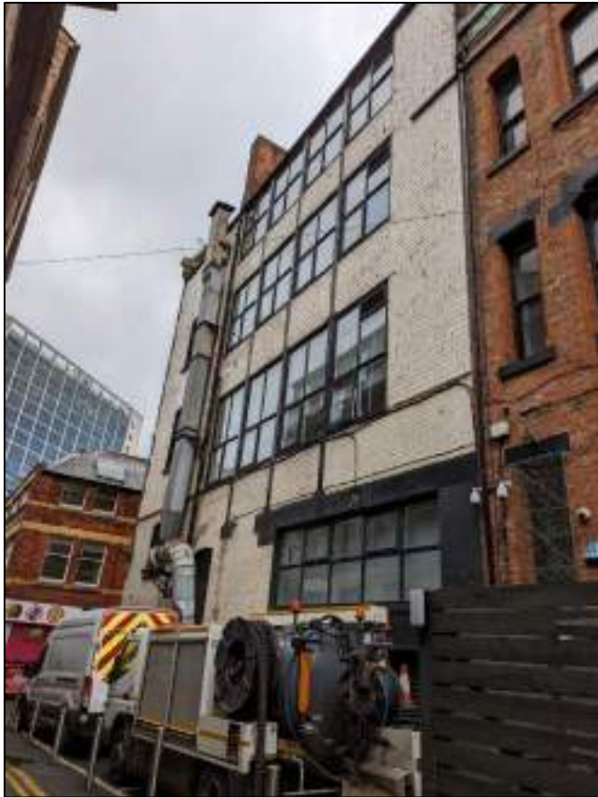
Plate 21: White glazed brick elevation of 1974 building
