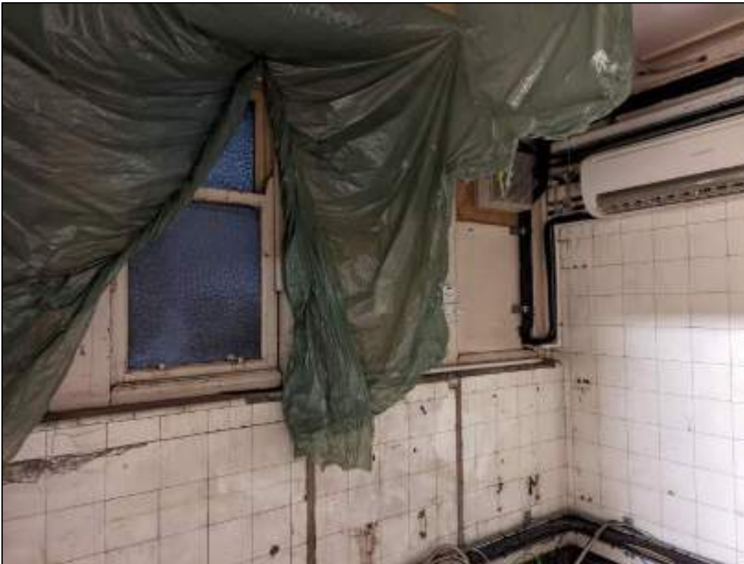
Plate 125: Stripped out toilet
