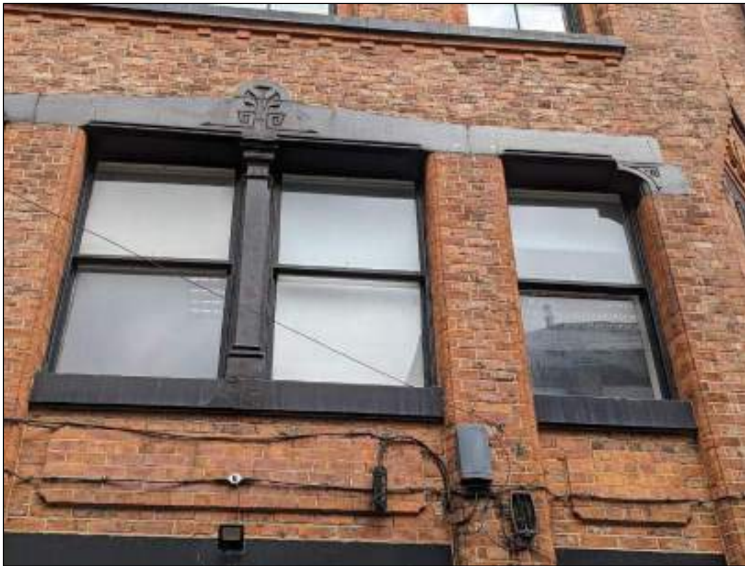
Plate 25: Detail of second floor windows
