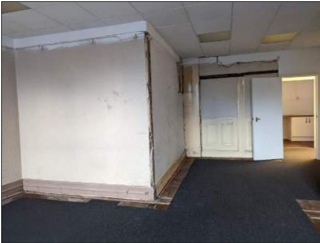
Plate 78: Stripped office space
