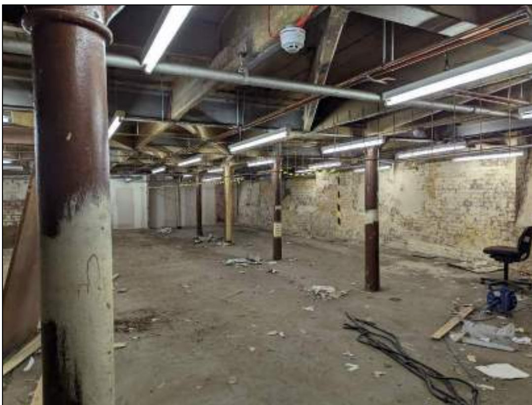
Plate 140: Large open room to west side of basement
