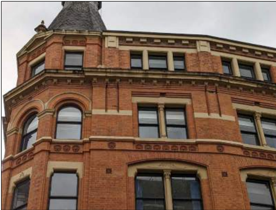
Plate 7: Detail of third and fourth floor windows
