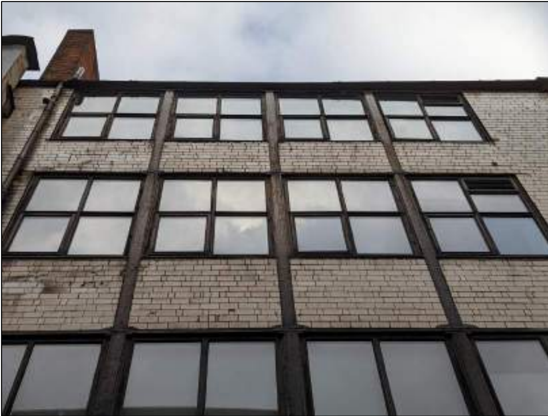
Plate 23: Upper floor windows
