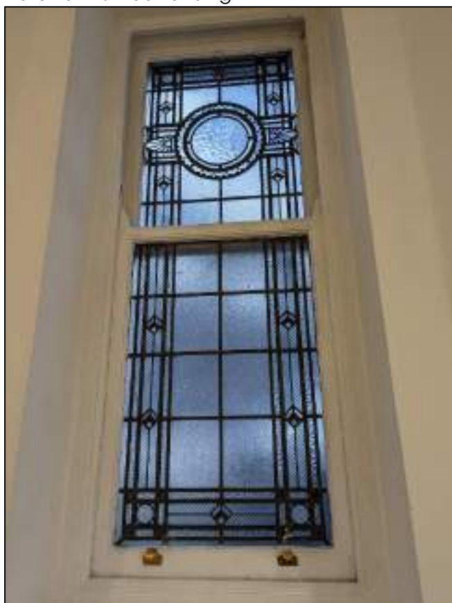
Plate 49: Detail of window on stairwell
