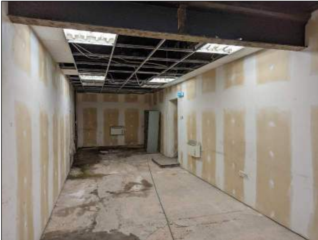
Plate 134: Rooms with plasterboard over walls
