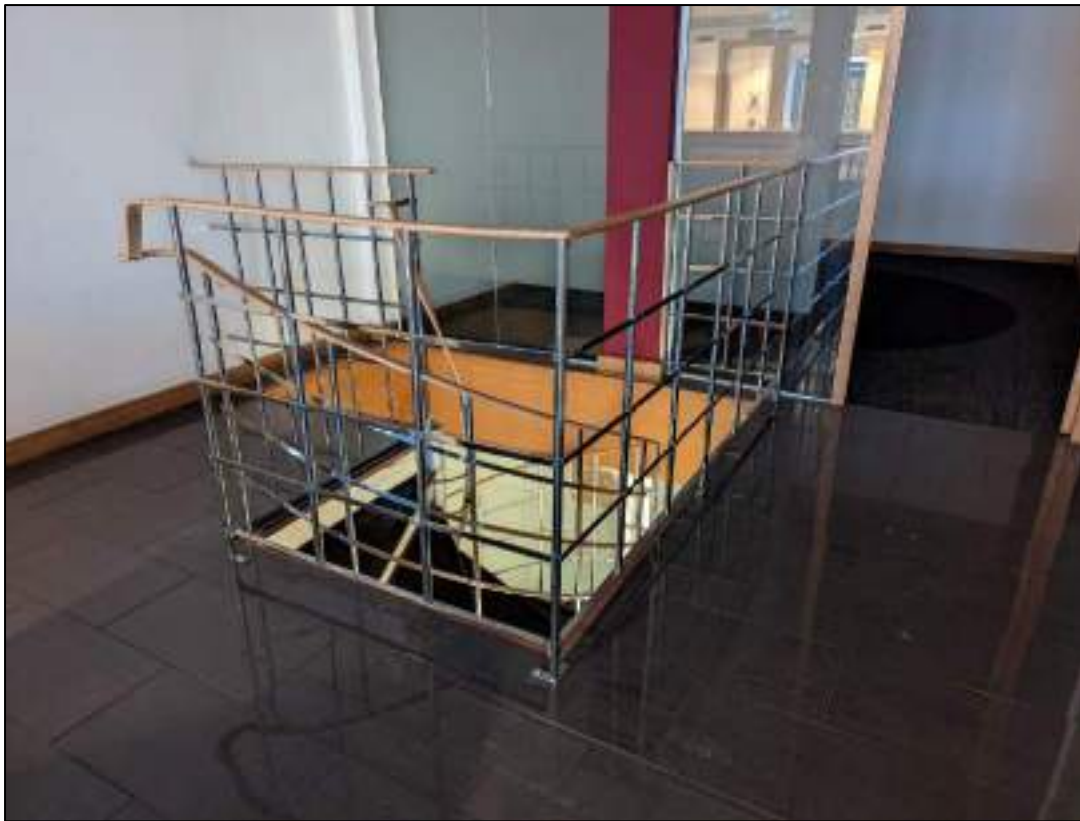
Plate 40: Inserted staircase to isolated upper basement
