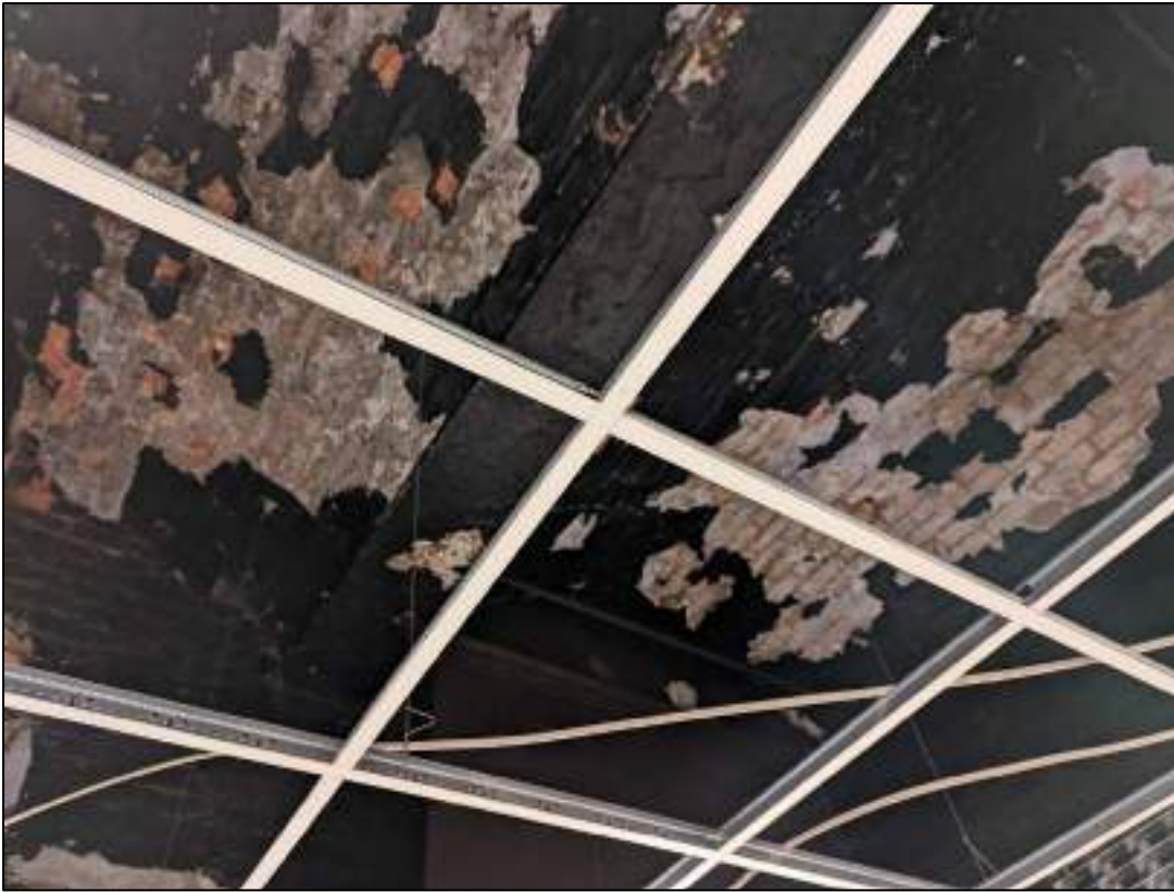
Plate 135: Brick vaulted ceiling on room above
