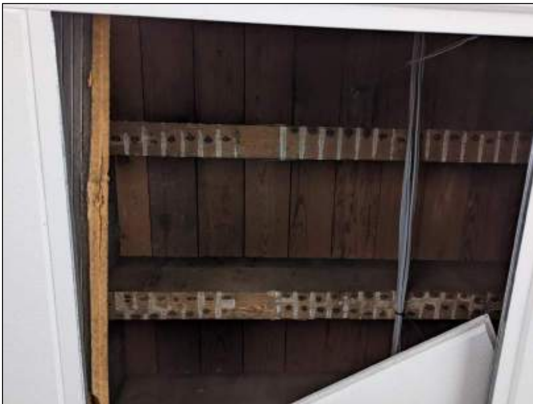
Plate 91: Revealed modern ceiling structure
