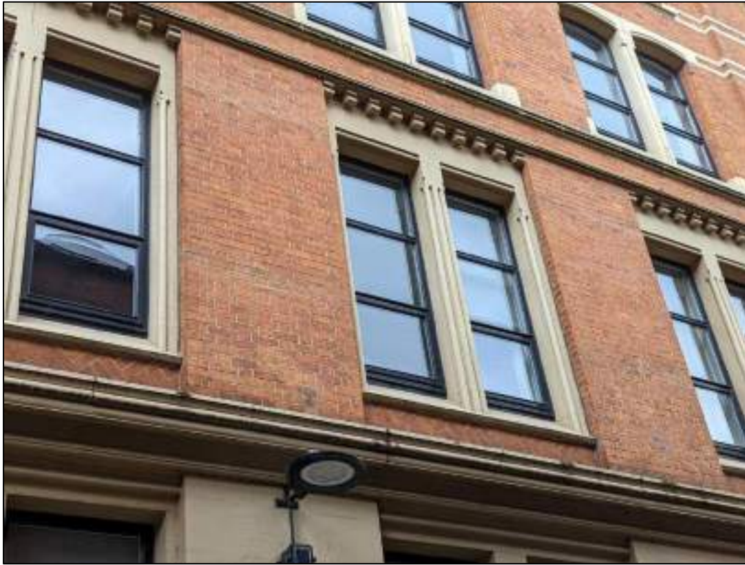
Plate 17: First floor window detail
