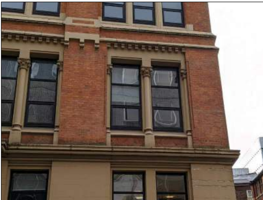
Plate 12: First floor windows of above
