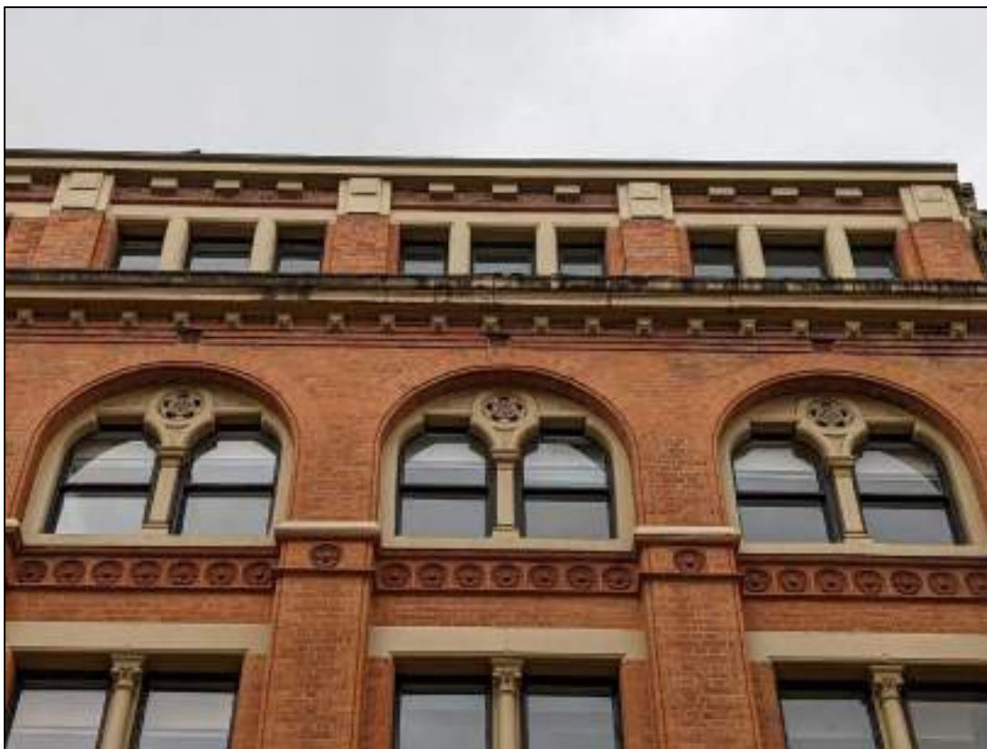
Plate 10: Third and fourth floor windows above hotel entrance
