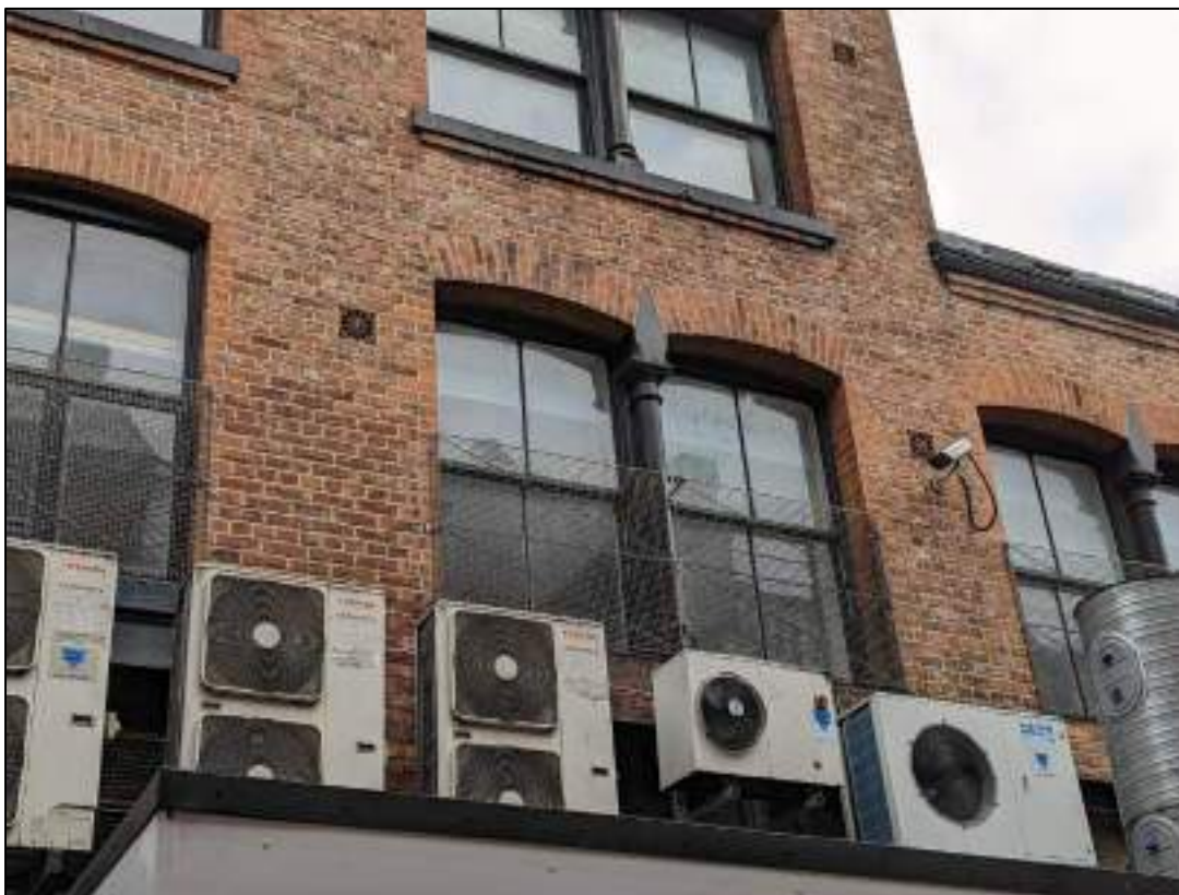
Plate 28: Upper floor windows of Household Stores building
