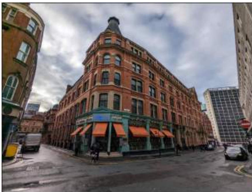
Image 1: Kings House - north and east elevations.
