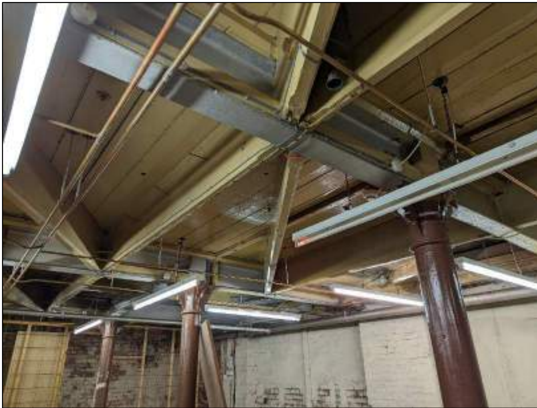
Plate 139: Timber ceiling detail
