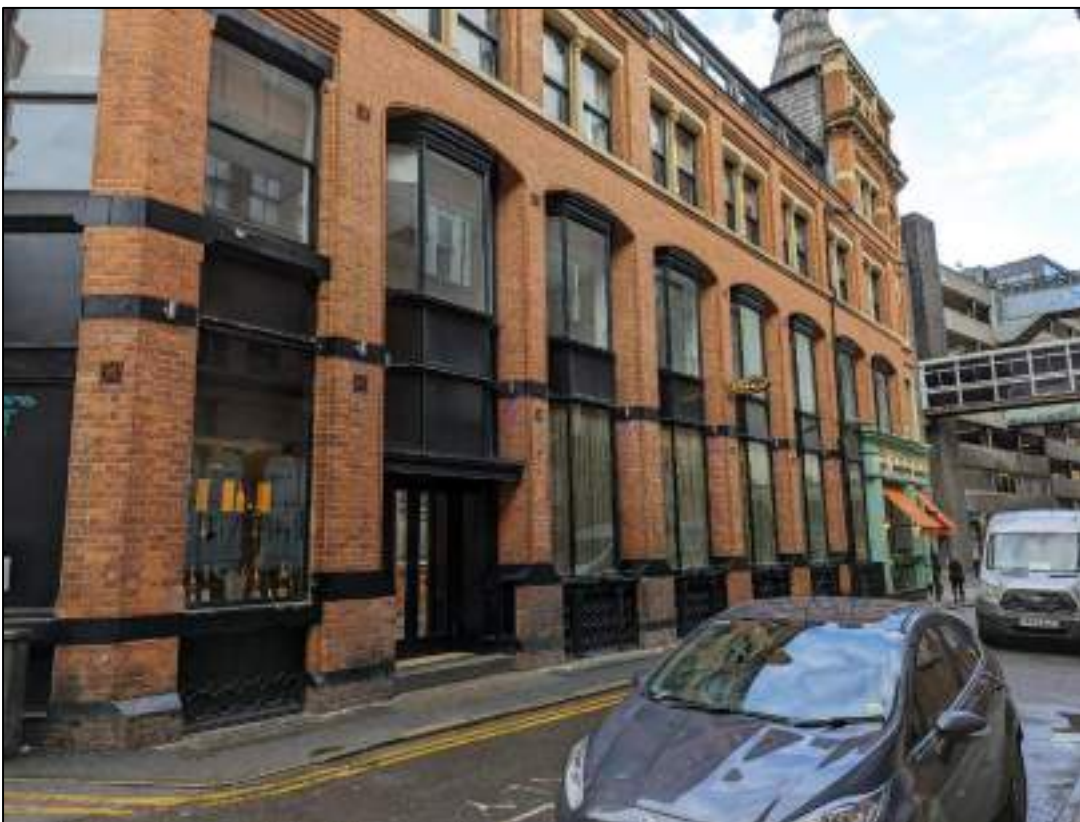
Plate 32: Ground and first floor windows
