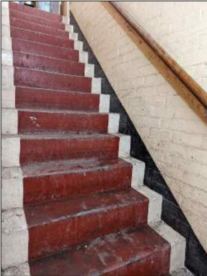
Plate 127: Staircase to Lower basement
