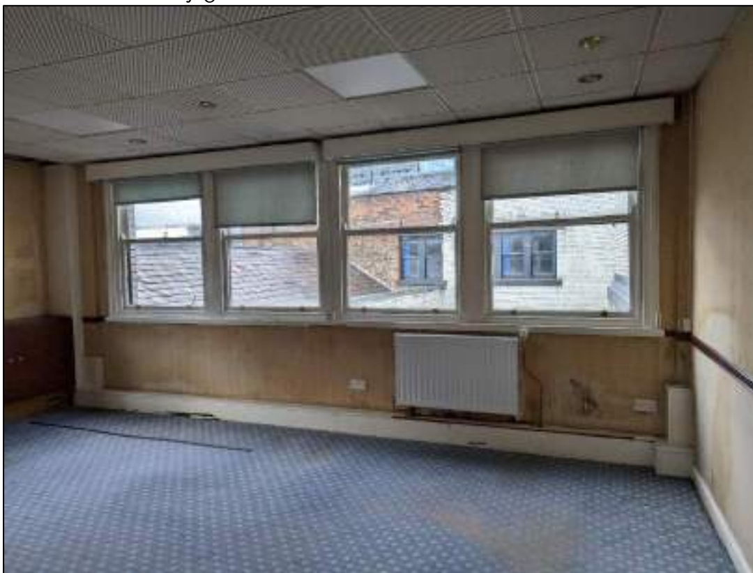
Plate 107: Long windows on fourth floor
