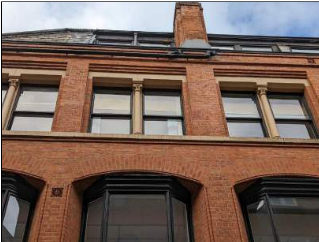
Plate 34: Detail of second and third floor windows
