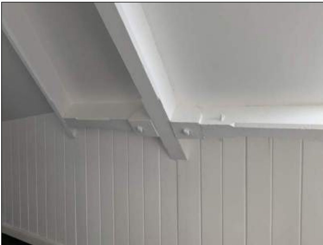
Plate 93: Timber roof structure
