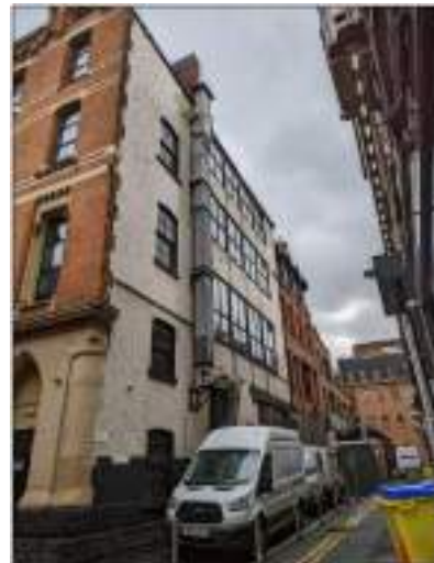
Image 5: Kings House – South elevation
