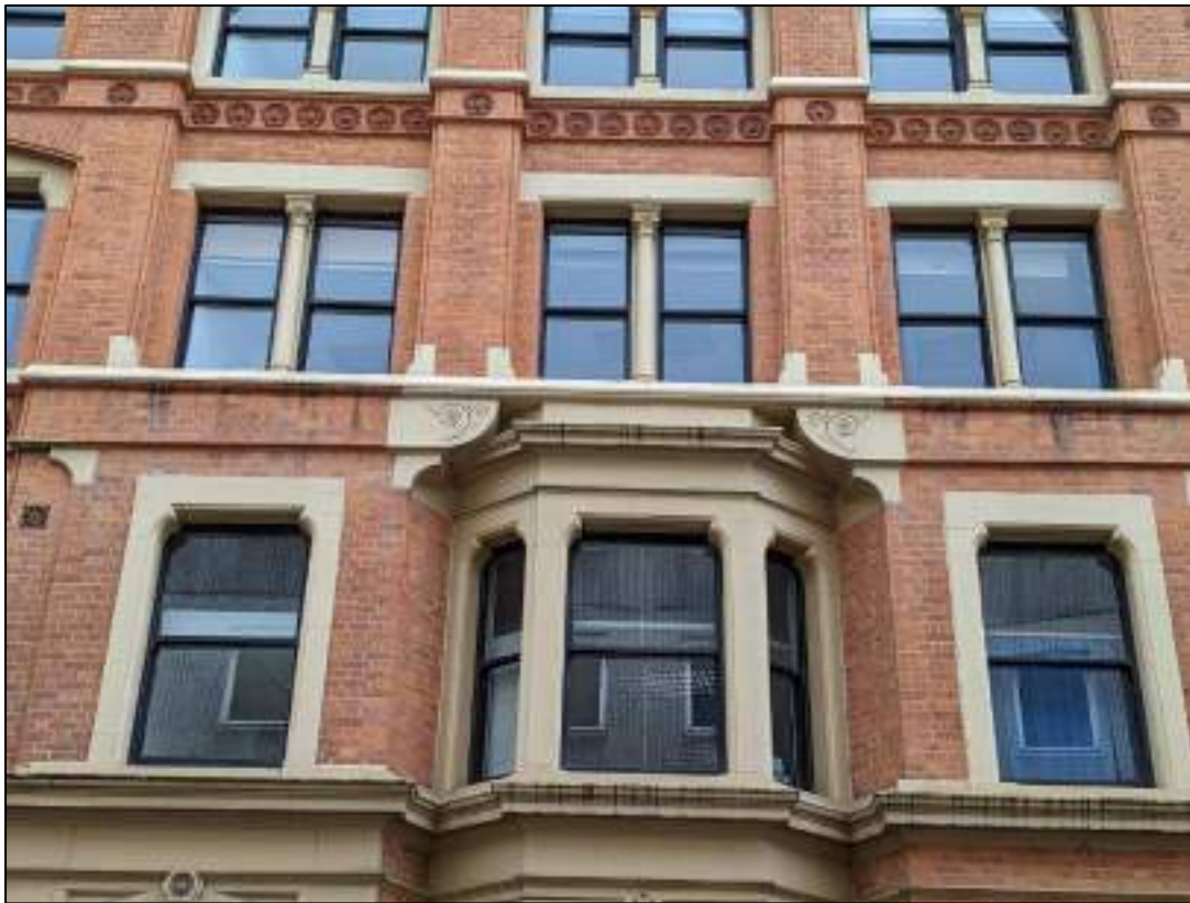
Plate 9: First and second floor windows above hotel entrance
