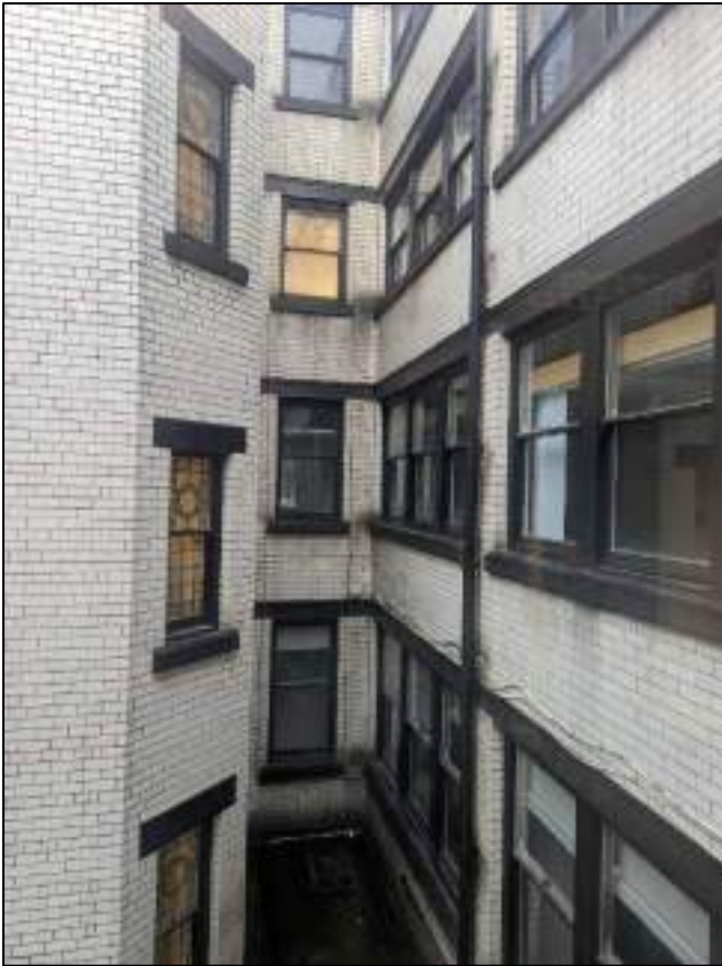
Plate 74: View of light well showing glazed brick
