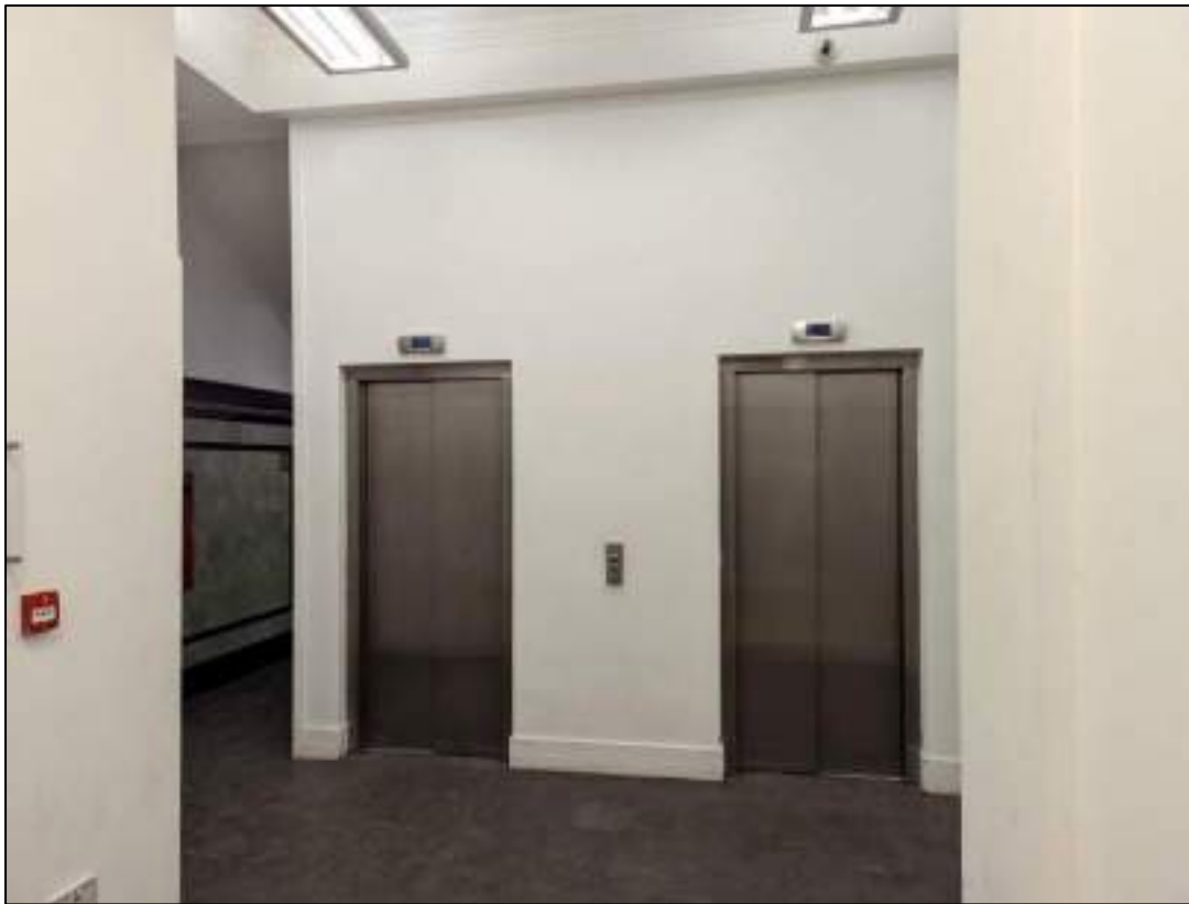
Plate 36: Entrance lobby with lifts
