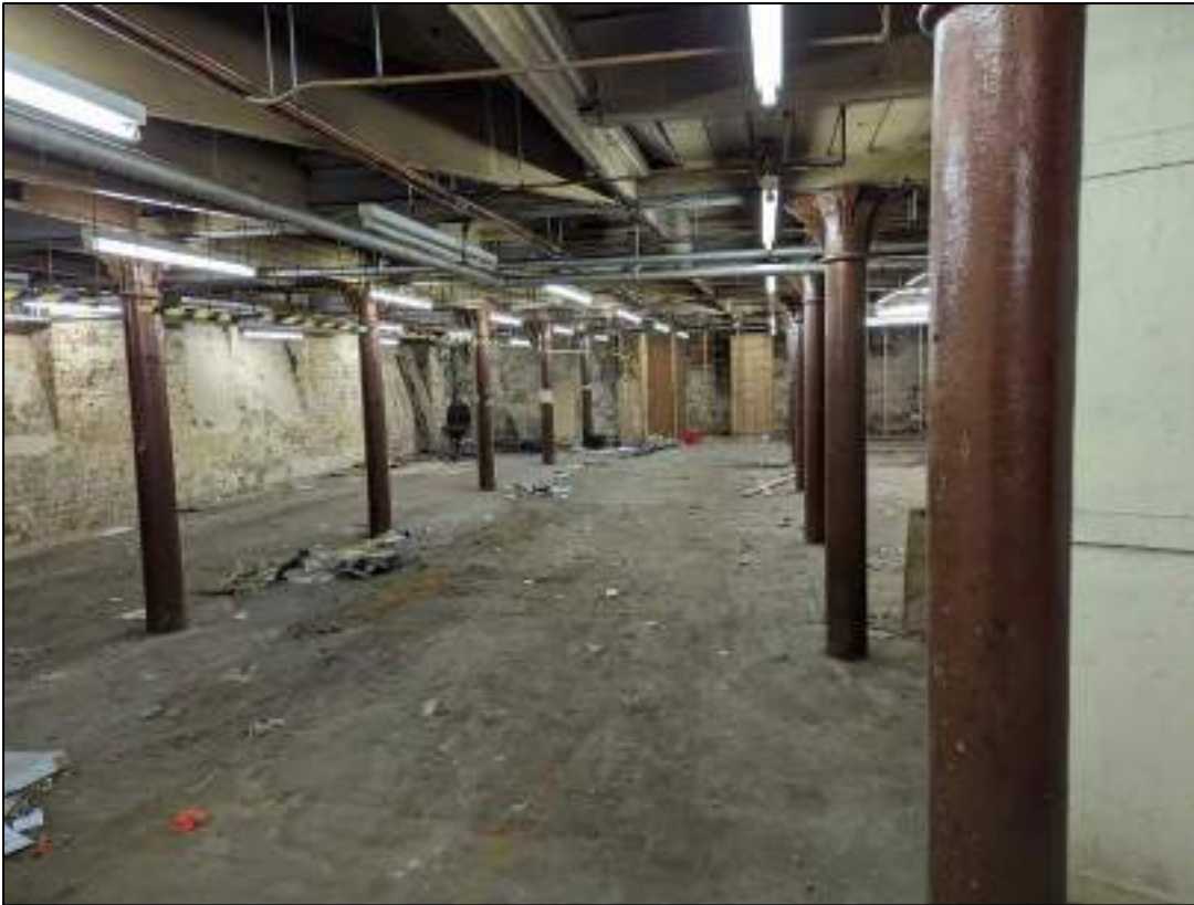
Plate 137: Large open room to west side of basement
