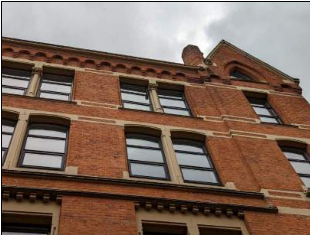
Plate 19: Upper floor windows towards Back Bridge Street
