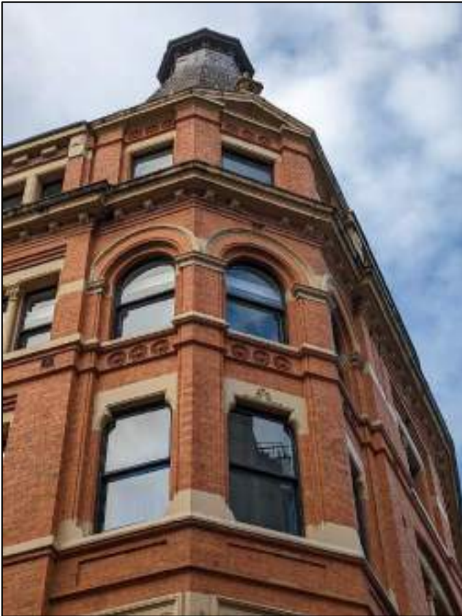
Plate 35: Upper floor windows of tower at corner with King Street West
