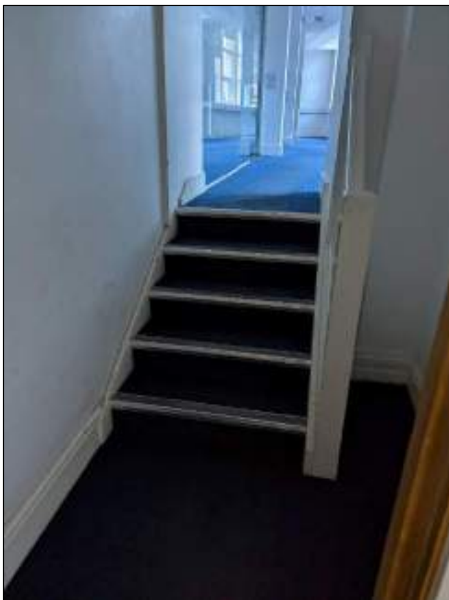
Plate 79: Staircase to 1974 building
