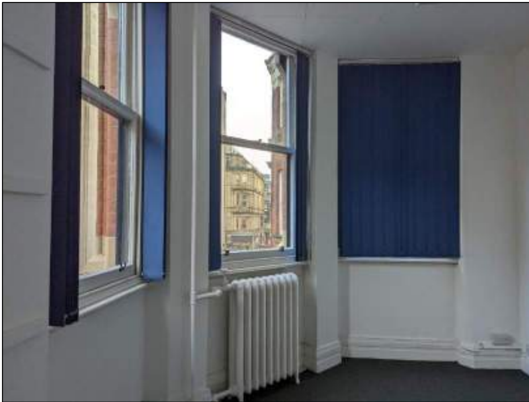
Plate 70: Windows to corner of King Street West and Southgate
