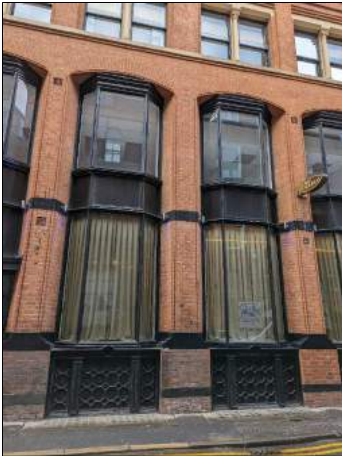
Plate 33: Detail of windows
