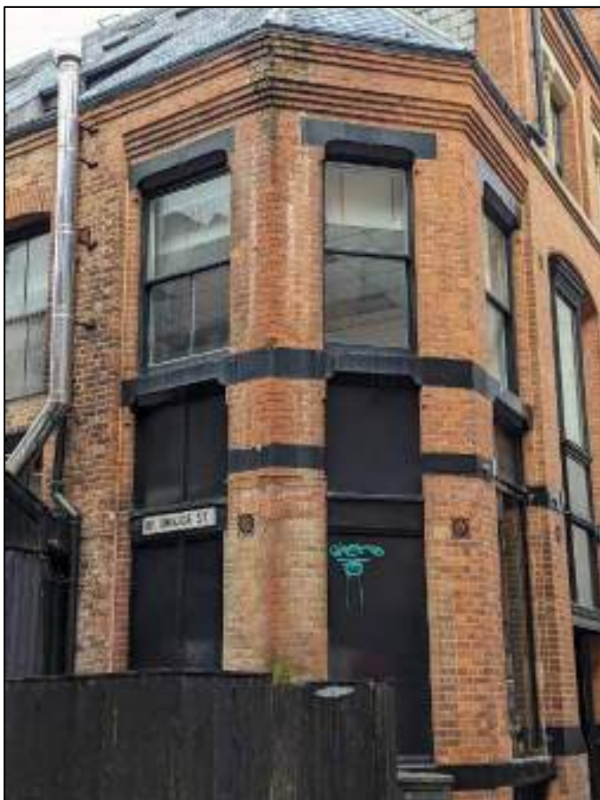
Plate 30: Ground floor windows at junction with Southgate
