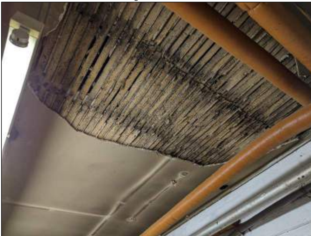
Plate 121: Revealed lath and plaster ceiling
