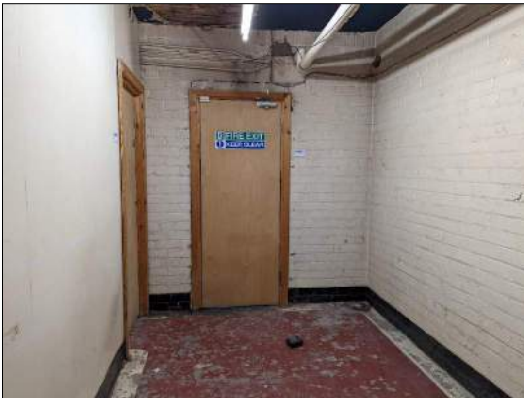
Plate 130: Inserted walls in basement
