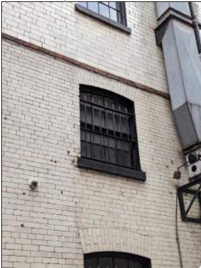
Plate 22: Detail of first floor window
