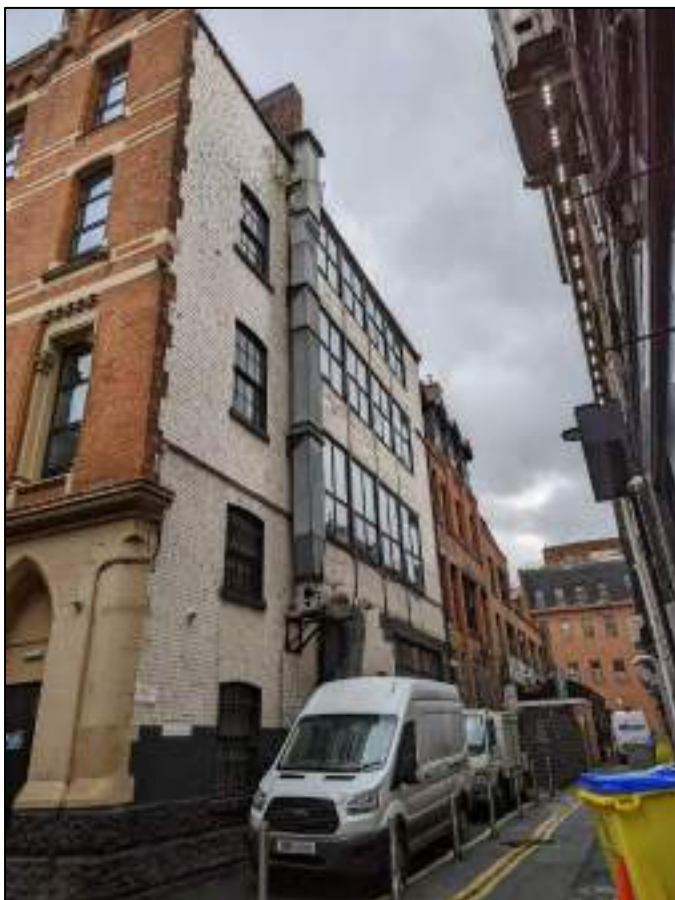
Plate 20: Back bridge street elevation
