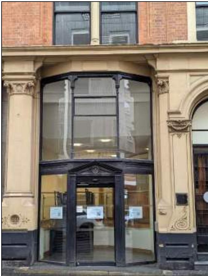
Plate 5: Inserted doorway in bay 6
