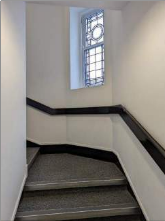
Plate 100: Staircase to fourth floor Fourth Floor
