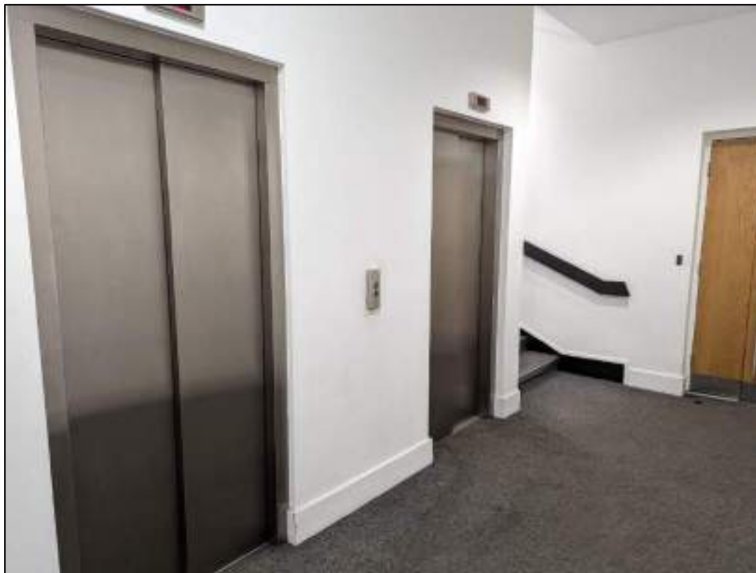
Plate 48: First floor landing
