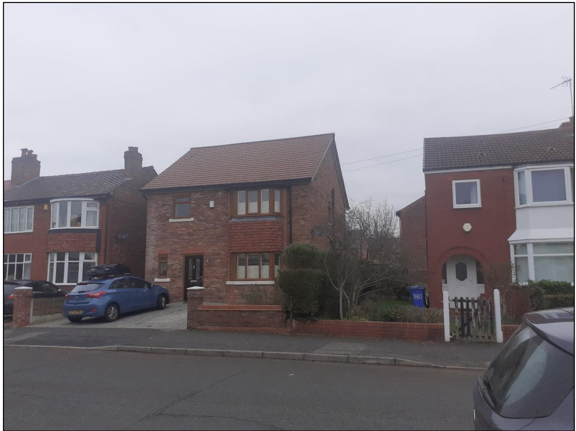
Figure 3: New dwelling constructed adjacent to 182 Manley Road.
