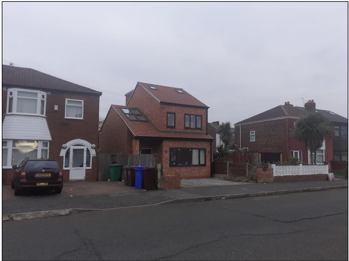
Figure 4: New dwelling constructed adjacent to 166 Manley Road.
