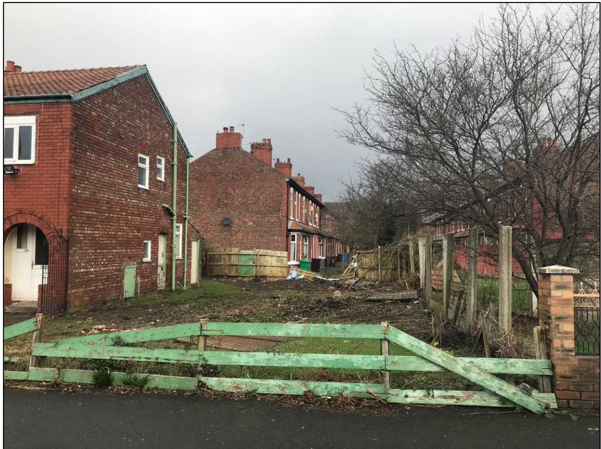
Figure 2: View of the site from Manley Road.
