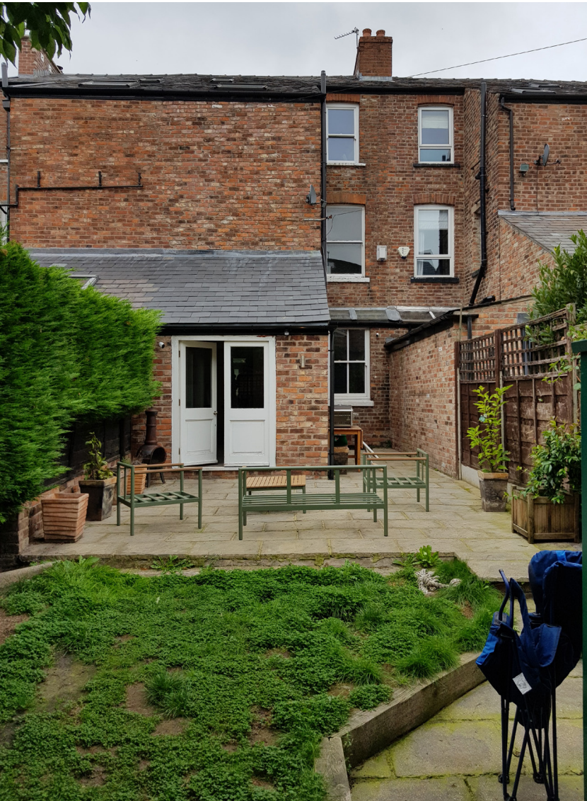
Current rear view of 39 Queenston Road
