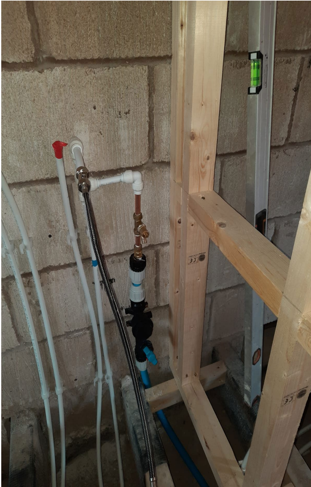
G. Internal new pipe work connection
