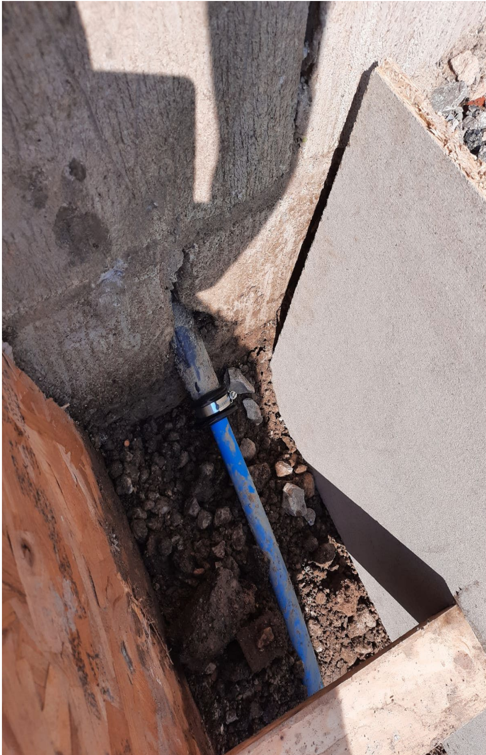
H. External new pipe work connection
