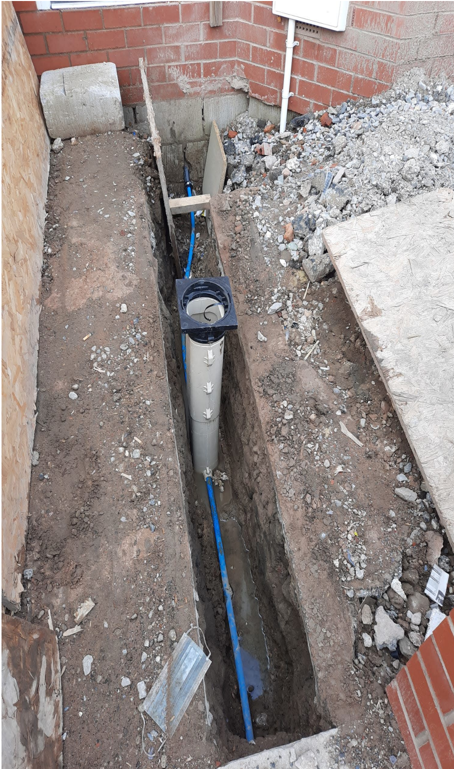
F. New below ground pipe works
