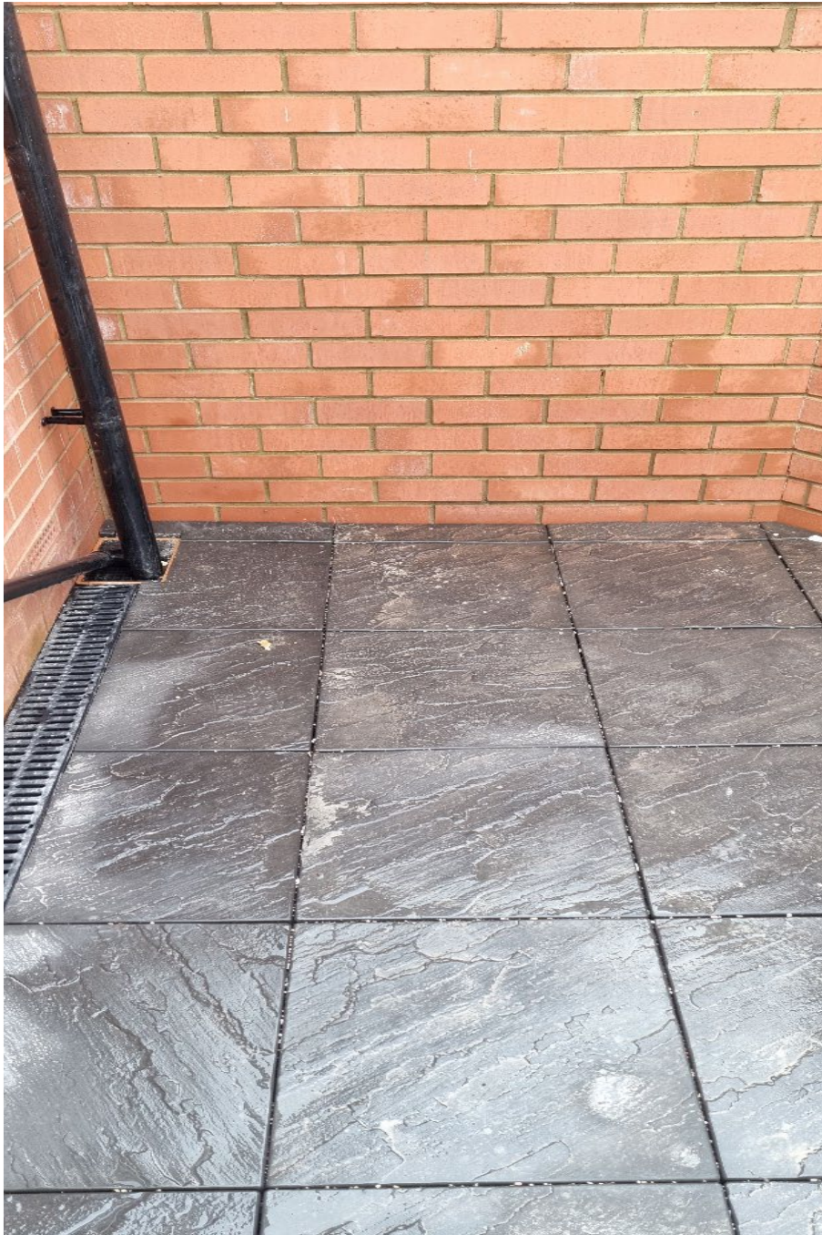
D. View of the new hard landscaping in the rear yard towards the house
