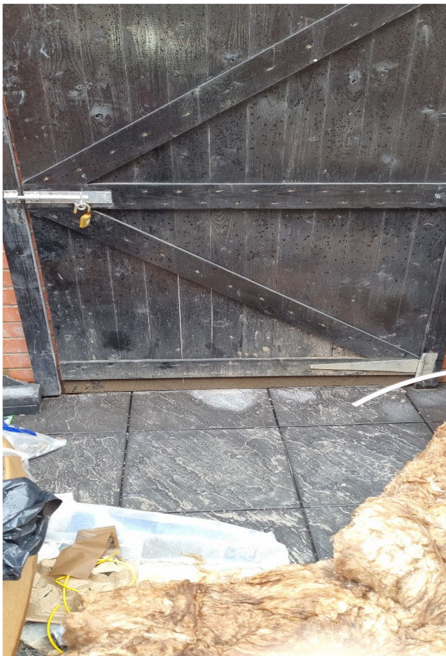
C. View of the new hard landscaping in the rear yard towards back gate
