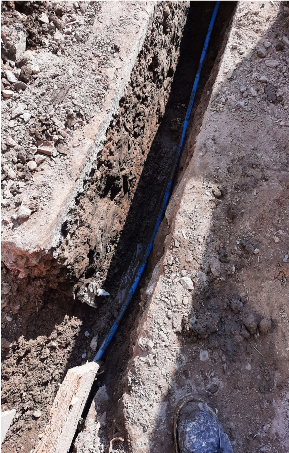
F. New below ground pipe works
