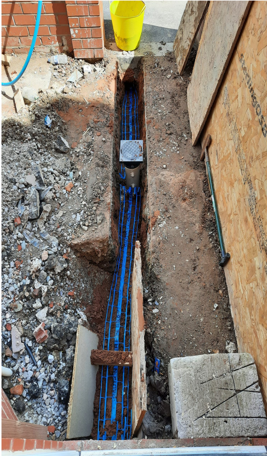
E. New below ground pipework
