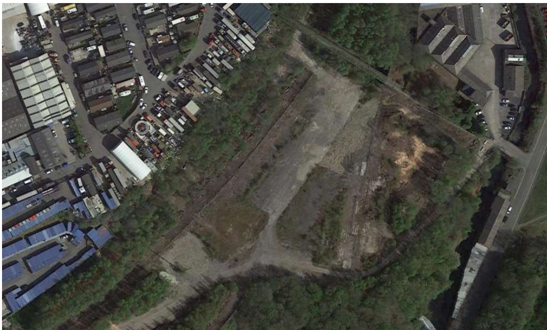
Figure 8: Extensive open hardstanding to north-eastern area of the site
