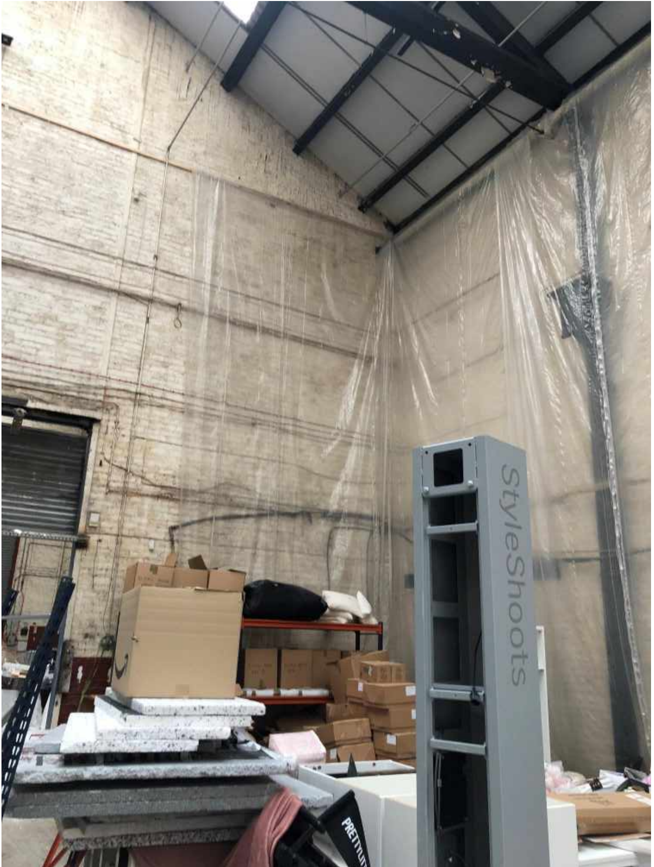
Photograph 9 Internal area of Ancoats Works, used for storage.
