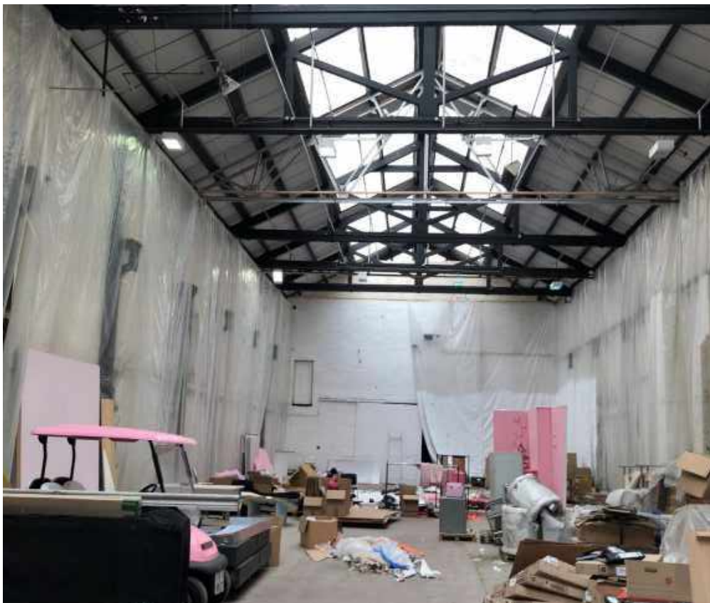
Photograph 14 Typical roof detail with plastic liner to walls of the large hall area.
