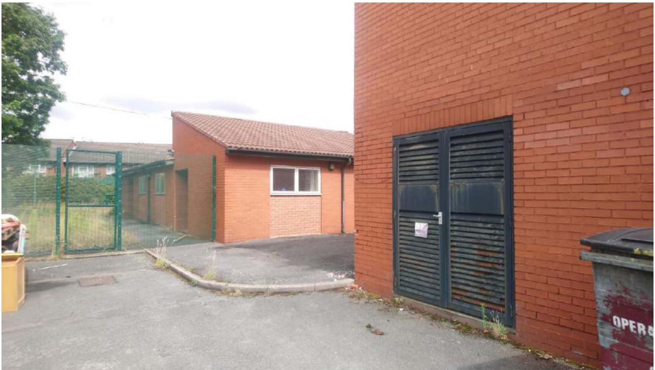
Photograph 2 View north-west towards a plant room on the southern elevation of the existing structure.
