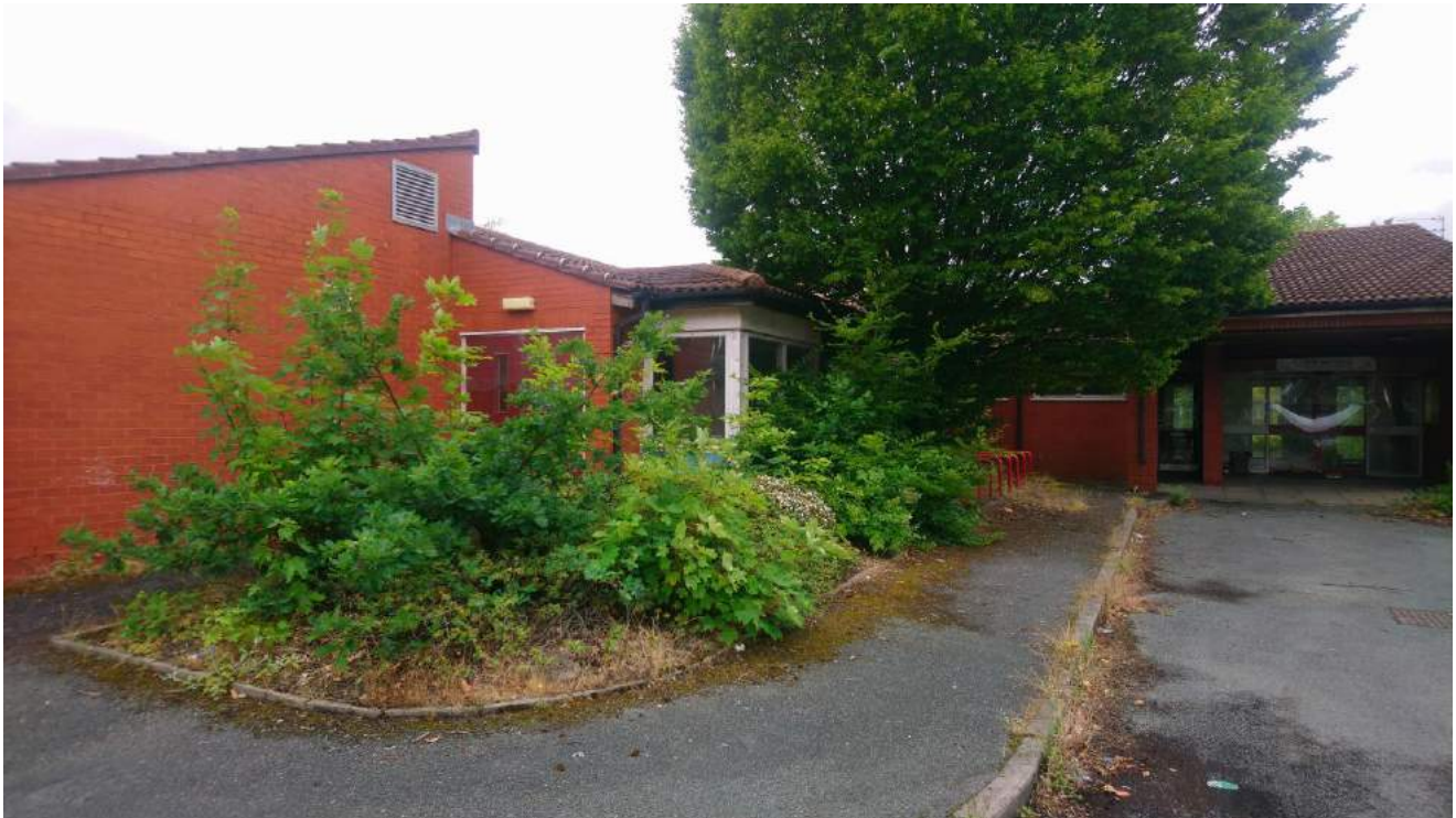
Photograph 1 View north towards the entrance to Oakwood Court in the central part of the site.
