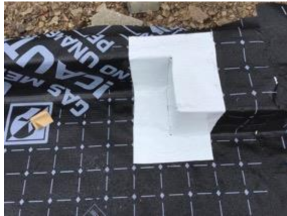
Plot 1 pipe seal with corner detail and patch repair using SAGM
