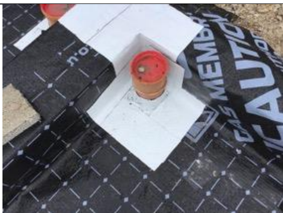
Plot 3 corner detail with pipe seal using SAGM
