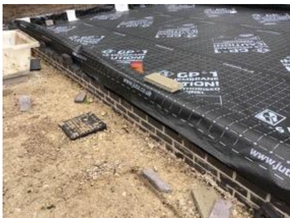
Plot 3 corner detail with pipe seal using SAGM
