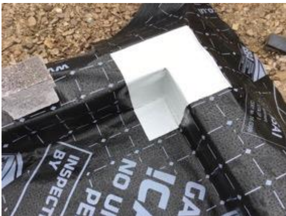
Plot 2 pipe seal using SAGM
