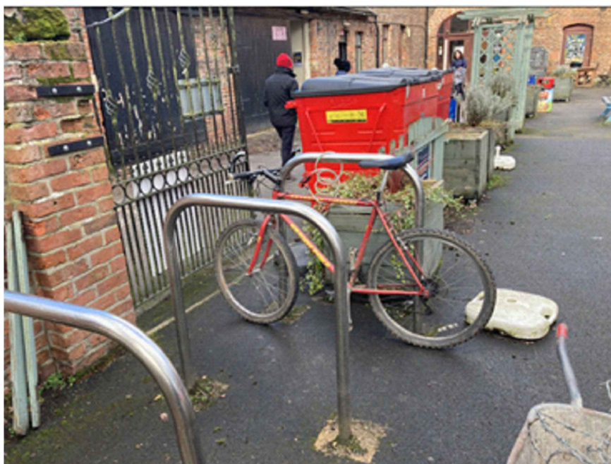
Photo 2: Existing cycle storage within Stables Courtyard comprising 3nr Sheffield stands; additional 4nr Sheffield stands to be provided. Total cycle storage provision of 7nr Sheffield stands.
