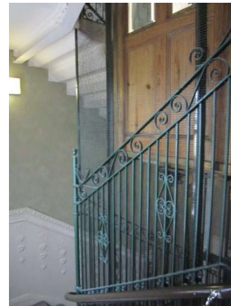
6 – Existing feature lift
