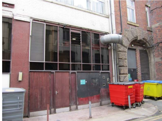
3 – View of rear of hotel – existing kitchen entrance
