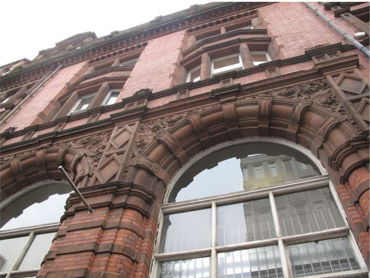
11. Details of 22 Dale Street (Grade II Listed)
