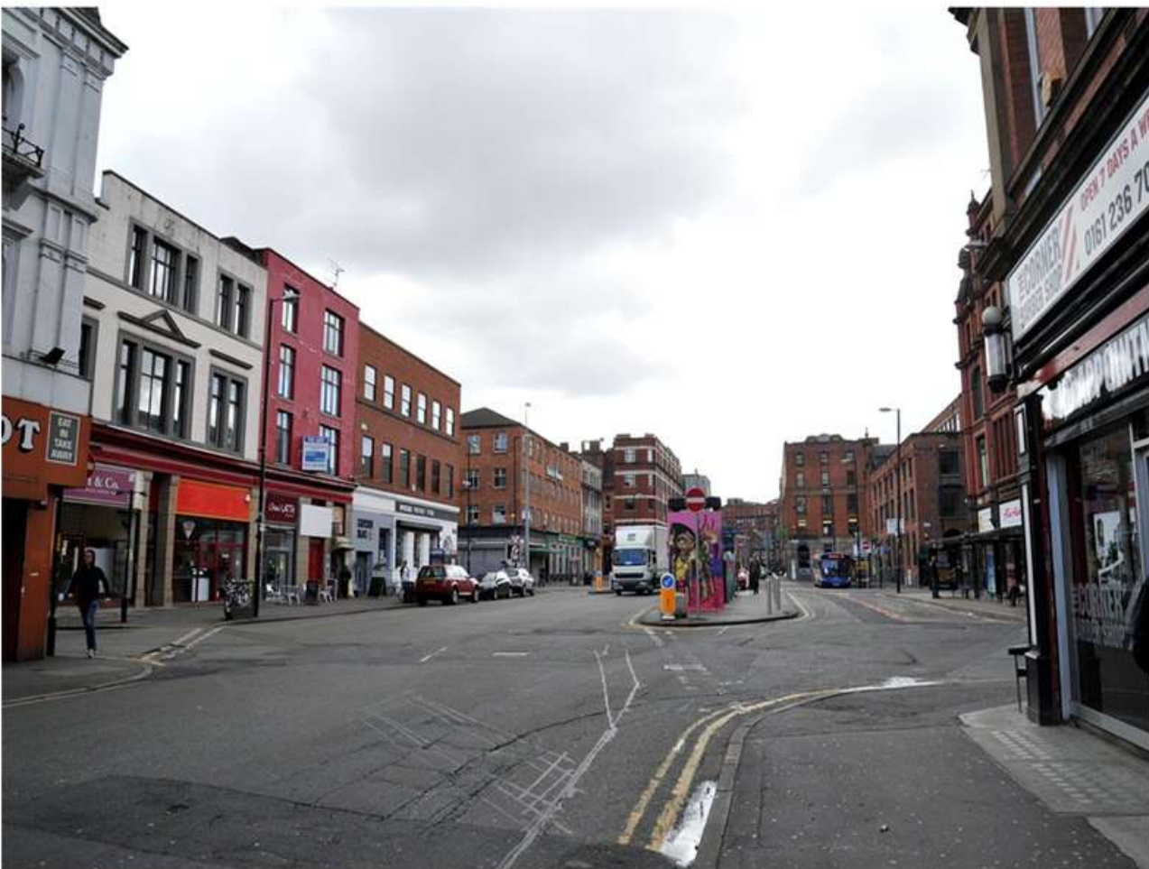
8. View of Stevenson Square from Hilton Street.
