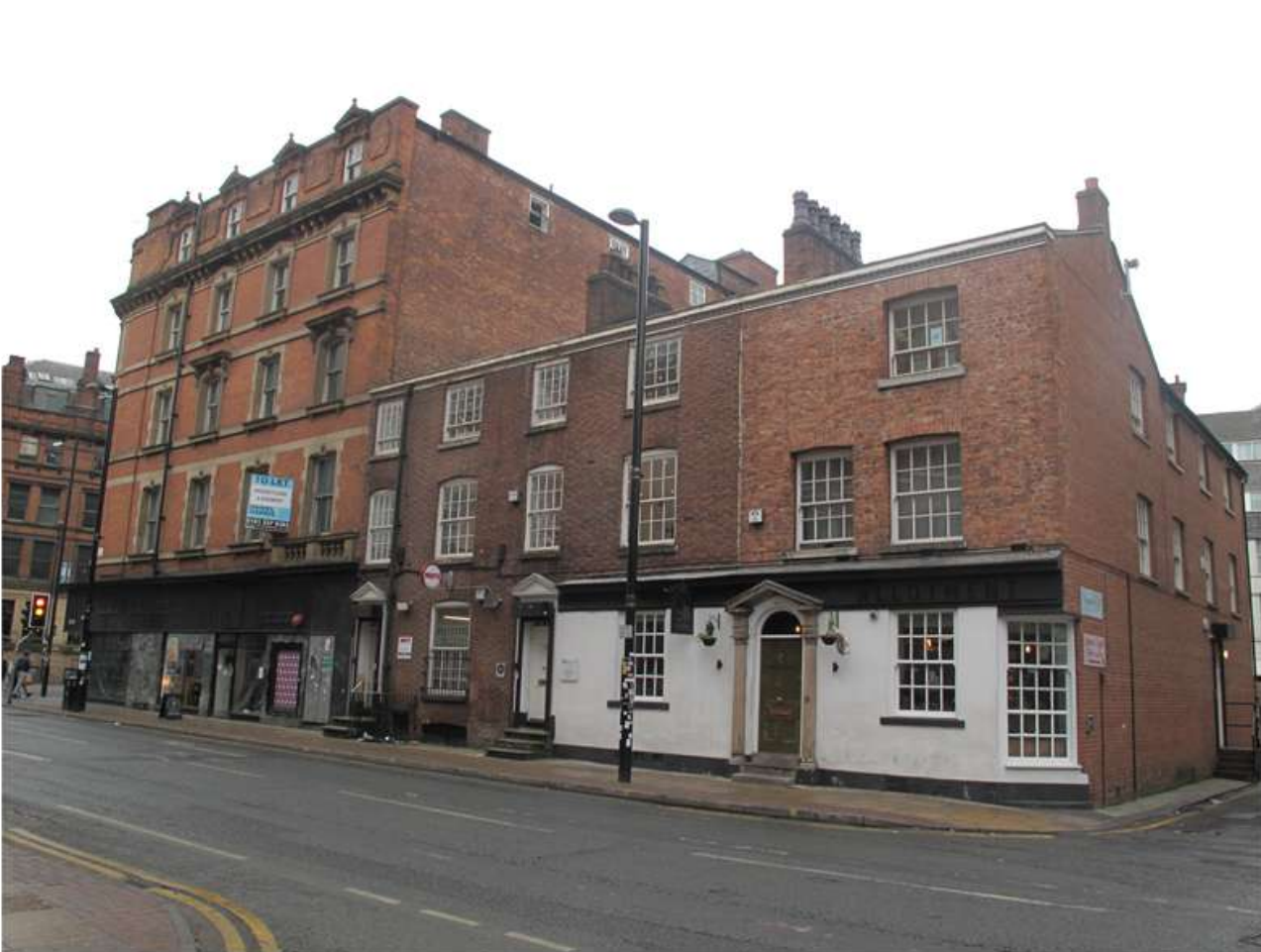
5. 32-34 Dale Street and Allotment Public House (both Grade II Listed).
