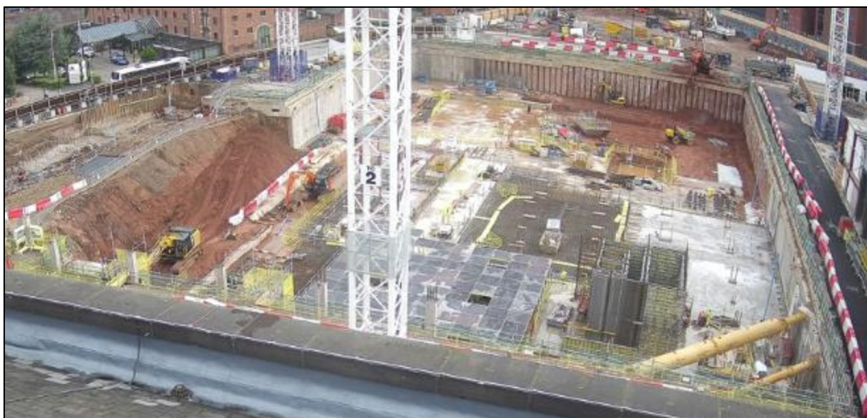
Photograph 6.3 Northern and Western extent of MGY excavation
