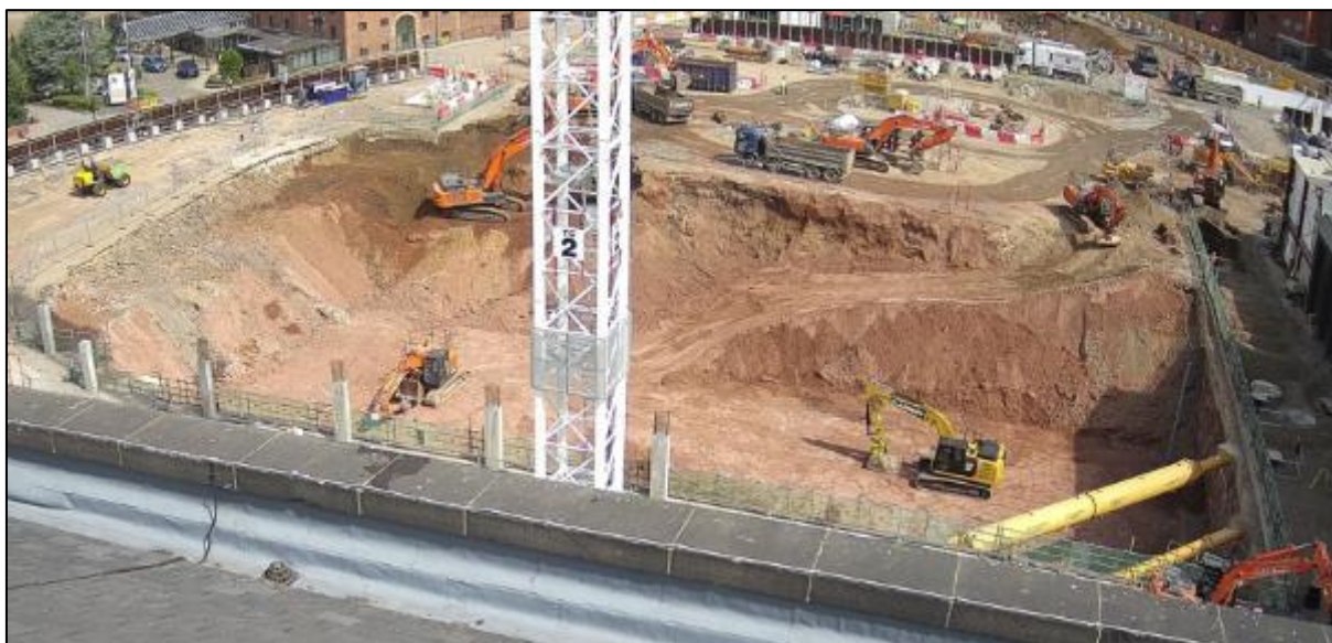
Photograph 6.1 Southern extent of MGY excavation
