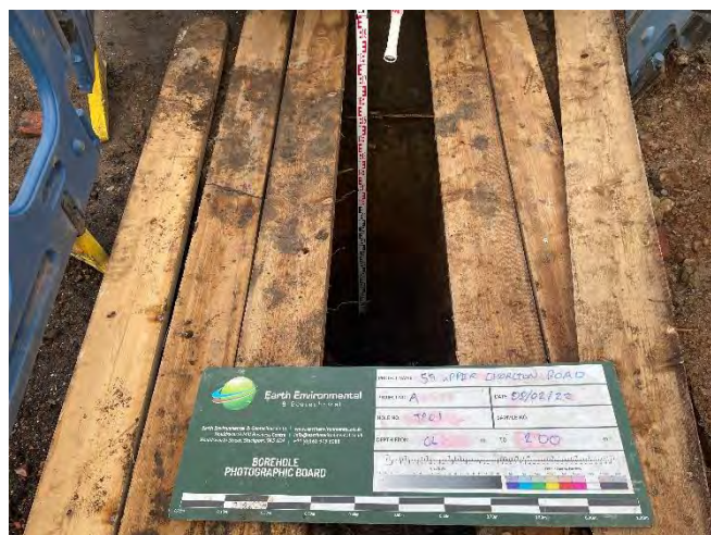
Soakaway Pit 1: Internal view of excavation
