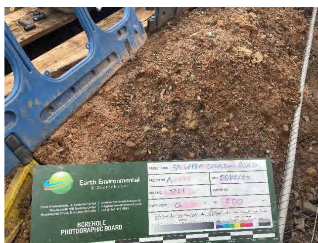
Soakaway Pit 1: Overview of excavated soils
