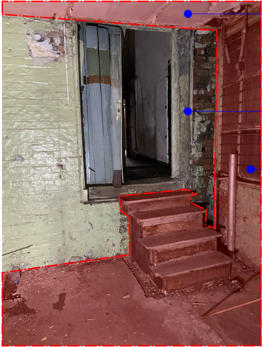
IMAGE 003- INTERNAL - Junction between retained and demolished - Warehouse
