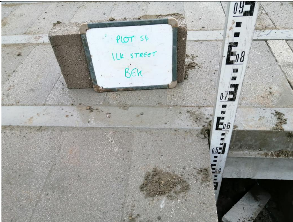
Photograph 3: Validation of Sub-Floor Void Space (min 150 mm)
