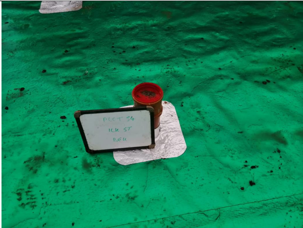
Photograph 7: Validation of Gas Membrane Installation
