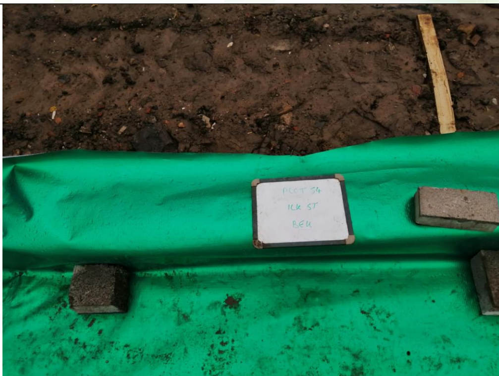
Photograph 8: Validation of Gas Membrane Installation
