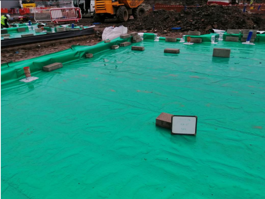
Photograph 5: Validation of Gas Membrane Installation
