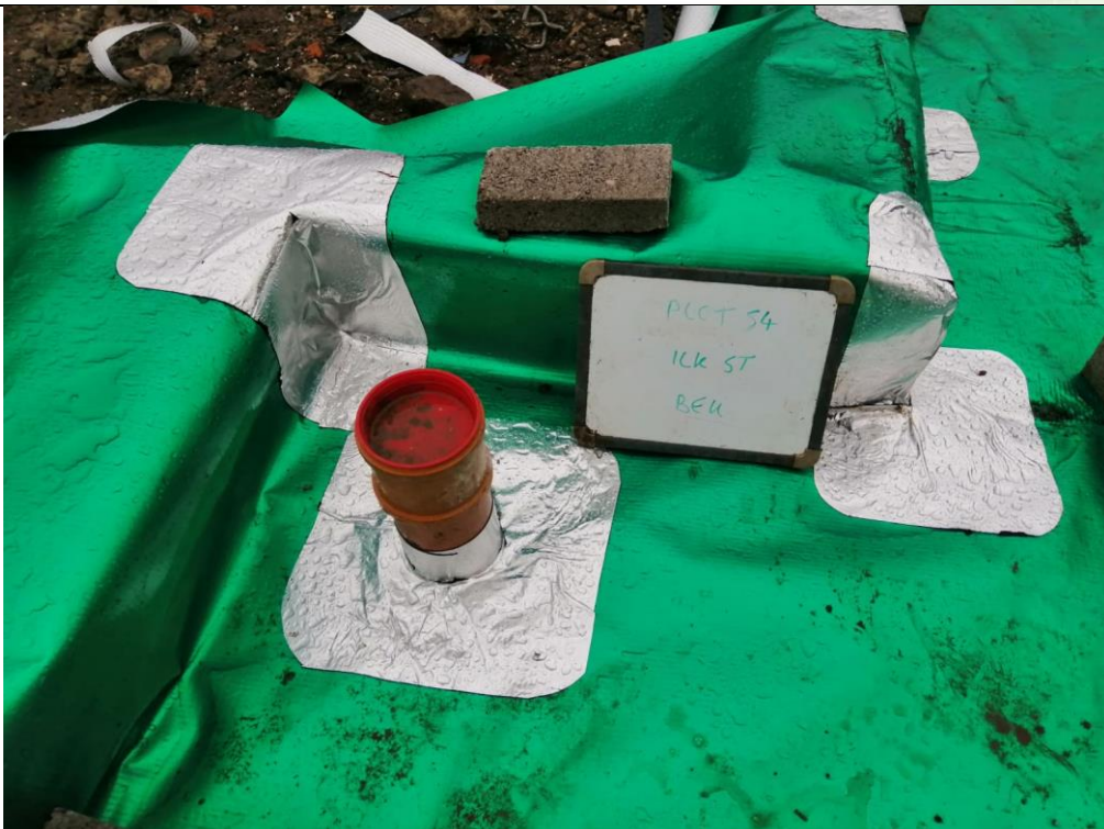
Photograph 6: Validation of Gas Membrane Installation
