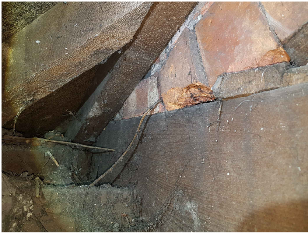
IMAGE 04: VIEW OF LEFT-HAND BEARING (AS VIEWED EXTERNALLY. SEE IMAGE 01) SHOWING TIMBER WEDGES AND CUT BRICK PACKERS TO AWKWARD TAPERED END OF RELIEVING ARCH, SIMILAR TO OPPOSITE BEARING (IMAGE 03). TIMBER BEAM APPEARS IN SOUND TIMBER CONDITION.
