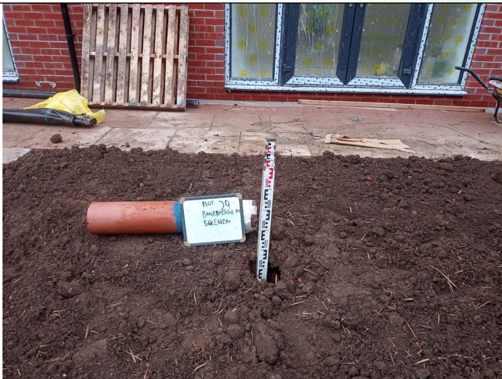
Photograph 2: Validation of Garden Capping Thickness
