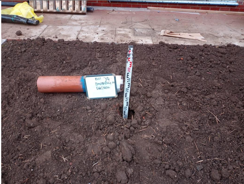
Photograph 1: Validation of Garden Capping Thickness
