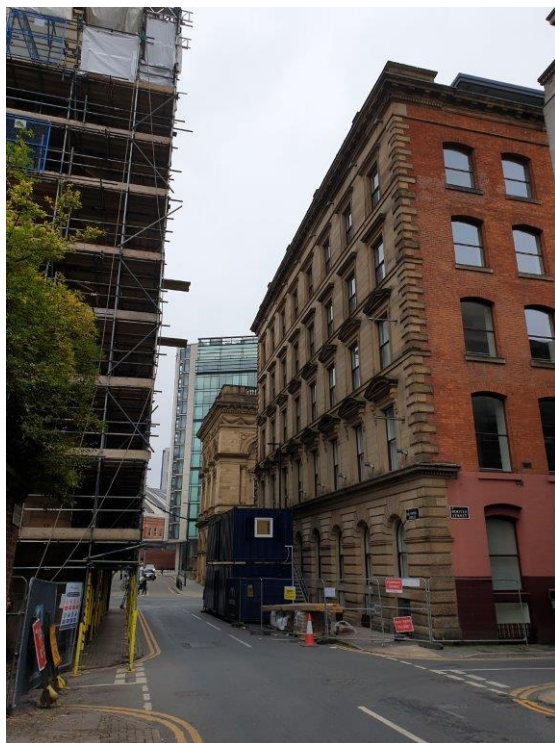
Image 4: Freetrade Exchange east elevation
