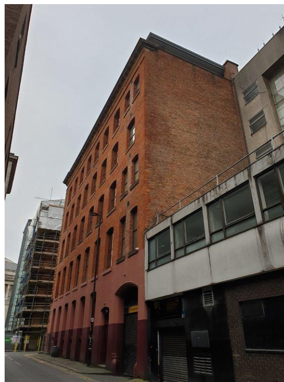
Image 5: North and visible part of west elevation
