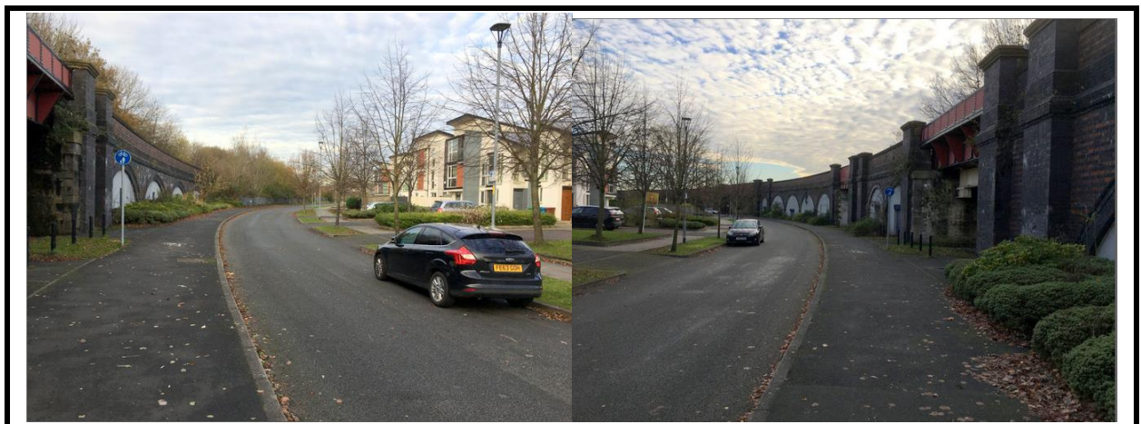
View from south and north approaches to cycle way under viaduct
