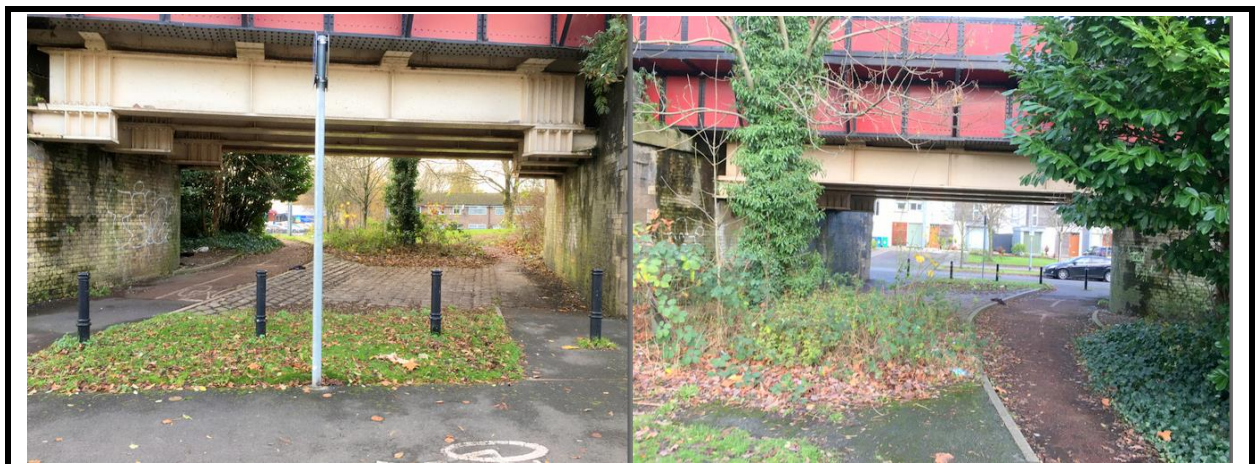
View west and east under viaduct route
