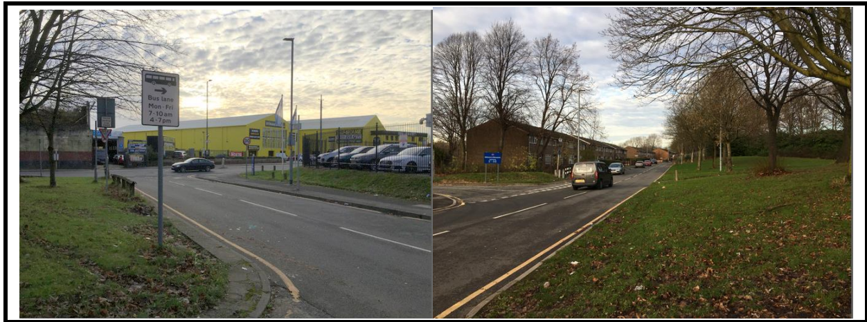
View left and right from site access
