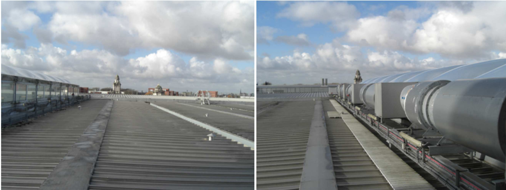
Above Left: View looking over ward 44 area, and the pitched standing seam roof. Right: View over ward 44 area showing existing large plant ducts.
