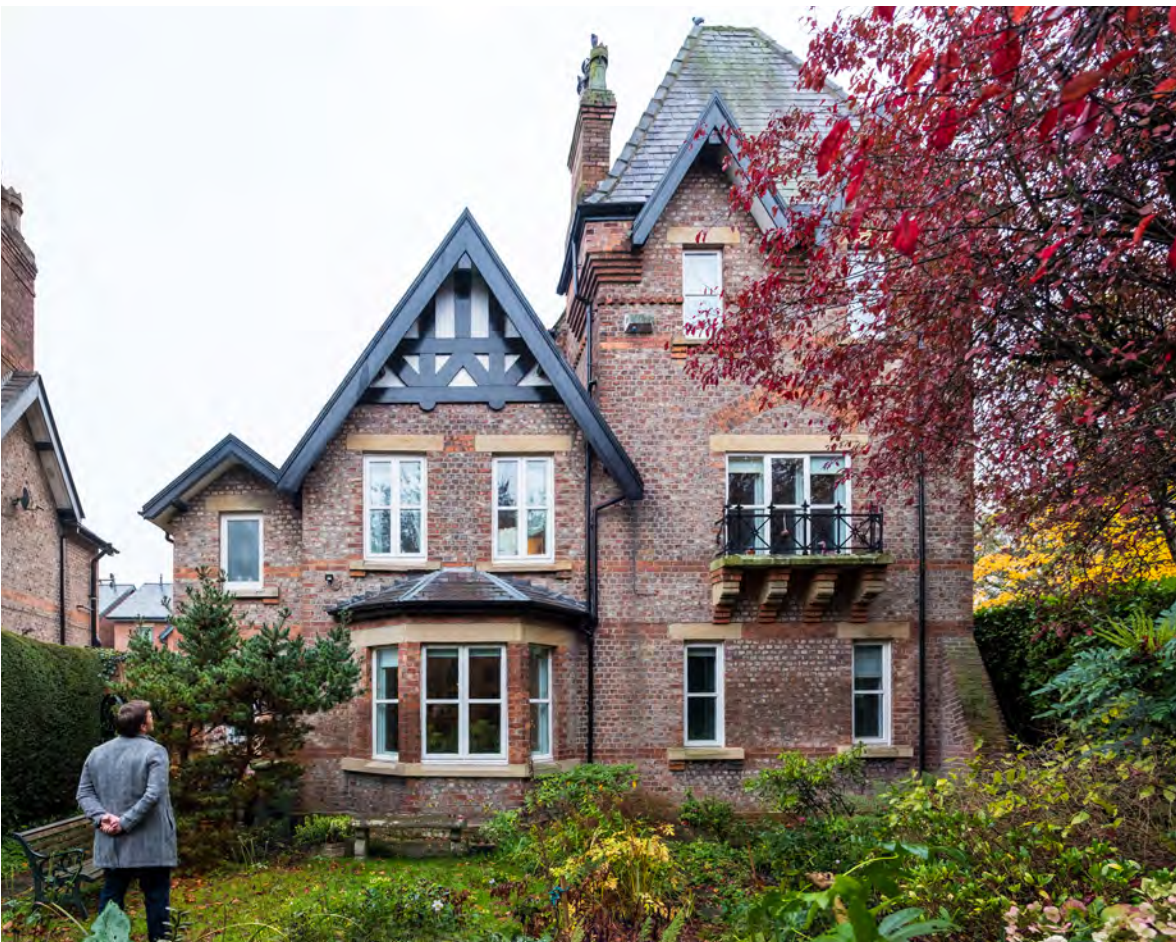
Figure 15 Photograph of Existing West Elevation
