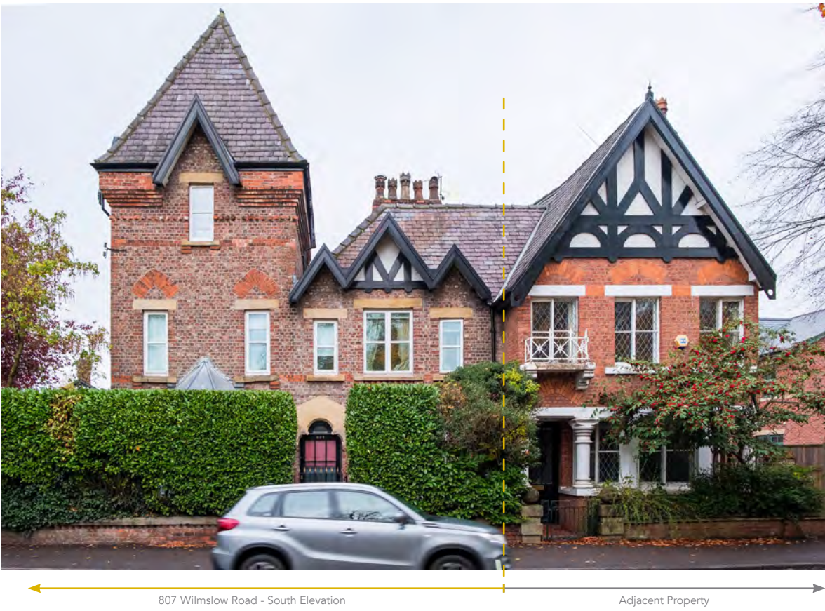
Figure 14 Photograph of South Elevation
