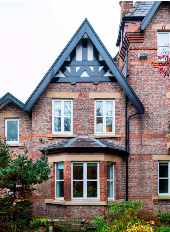
Existing West Elevation Photograph Not to Scale
