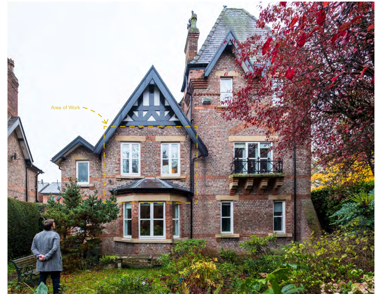
Figure 3 Photograph of Existing West Elevation, with the area of work highlighted
