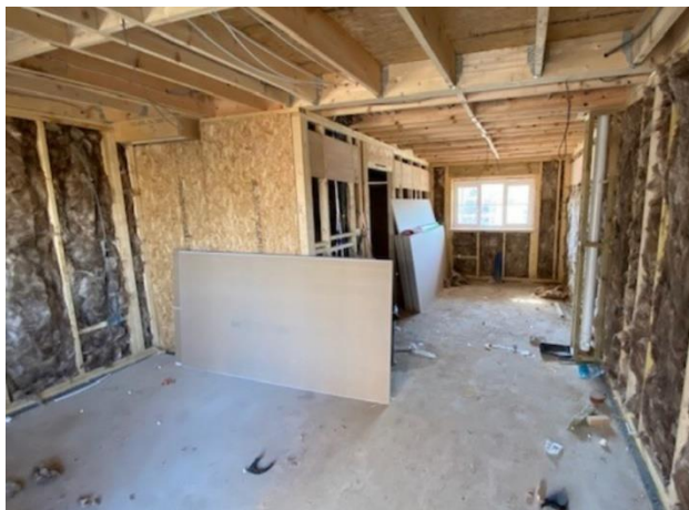
Photograph showing insulation installed to the internal studs of the timber frame on external elevations and party wall. Photograph taken April
