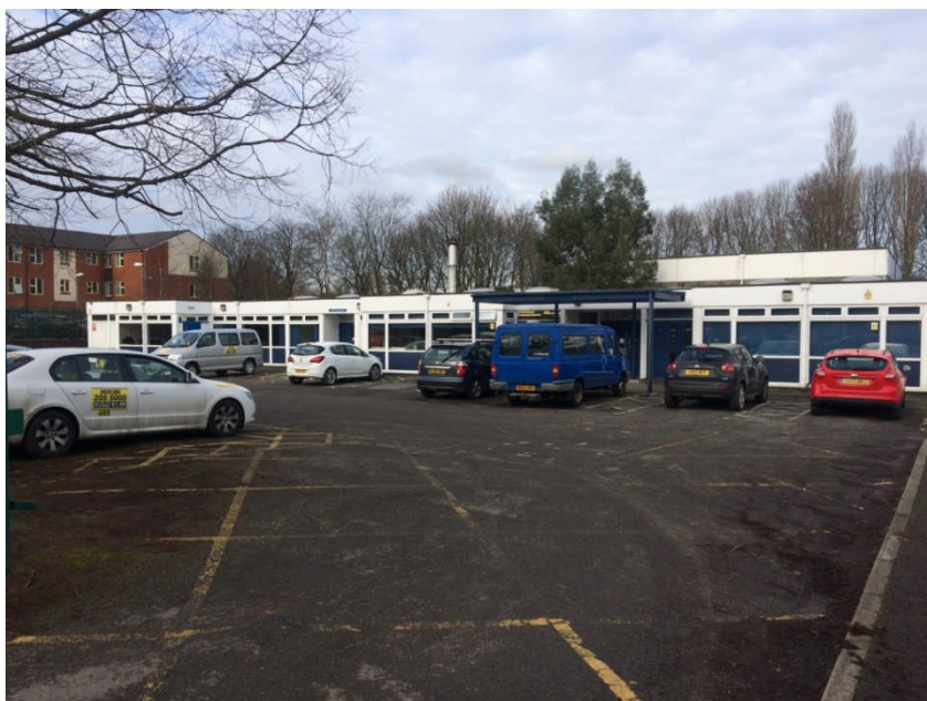
Photo 10: View north showing front elevation of B1 and large car park. Eucalyptus tree within enclosed courtyard is visible above the roof line (centre).
