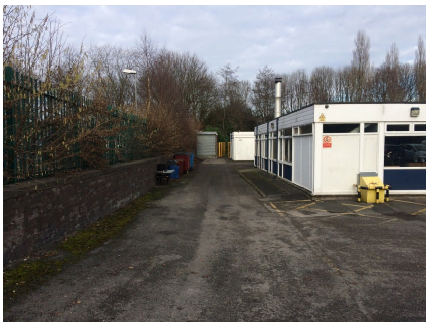
Photo 2: View north along western site boundary, showing western end of B1, with the grey roller door of B7 garage visible in the distance.
