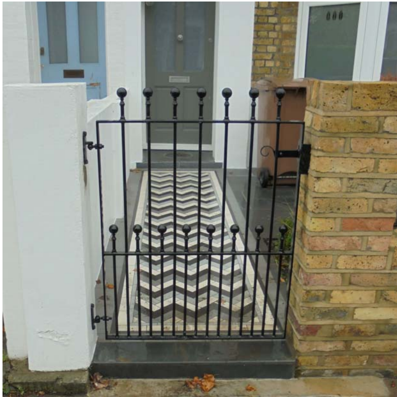
Facing brickwork, size, colour mix and cut to match existing.
