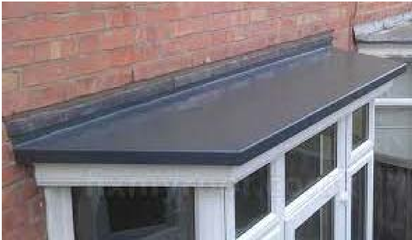
Warm roof with IKO Ruberseal EPDM or GRP high performance single ply roofing membrane on Kingspan TR27 Insulation.
