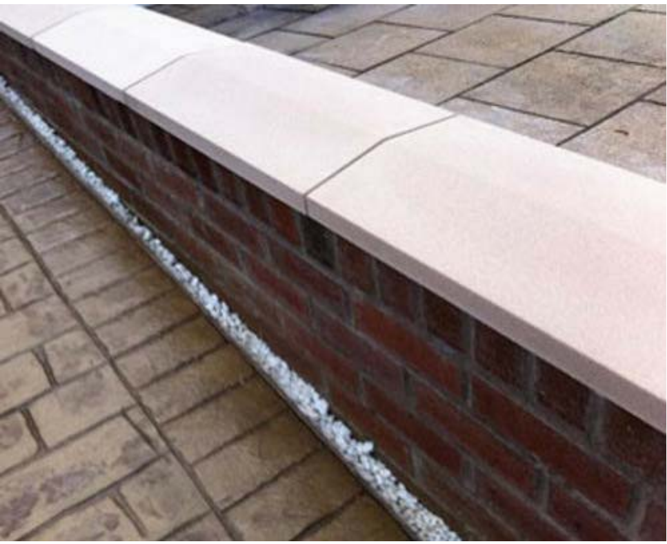
Facing brickwork, size, colour mix and cut to match existing.
