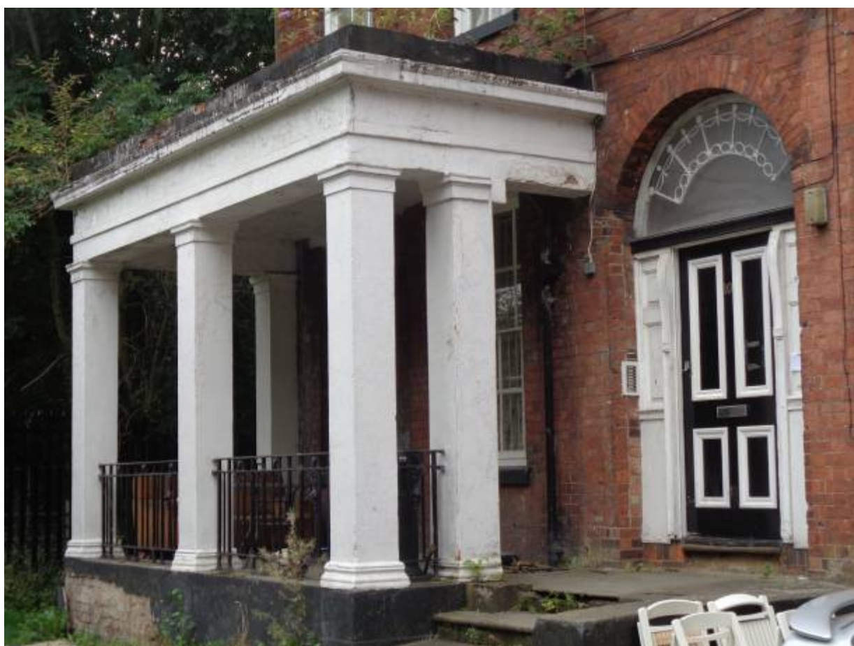
3. Unusual loggia by the entrance, probably later
