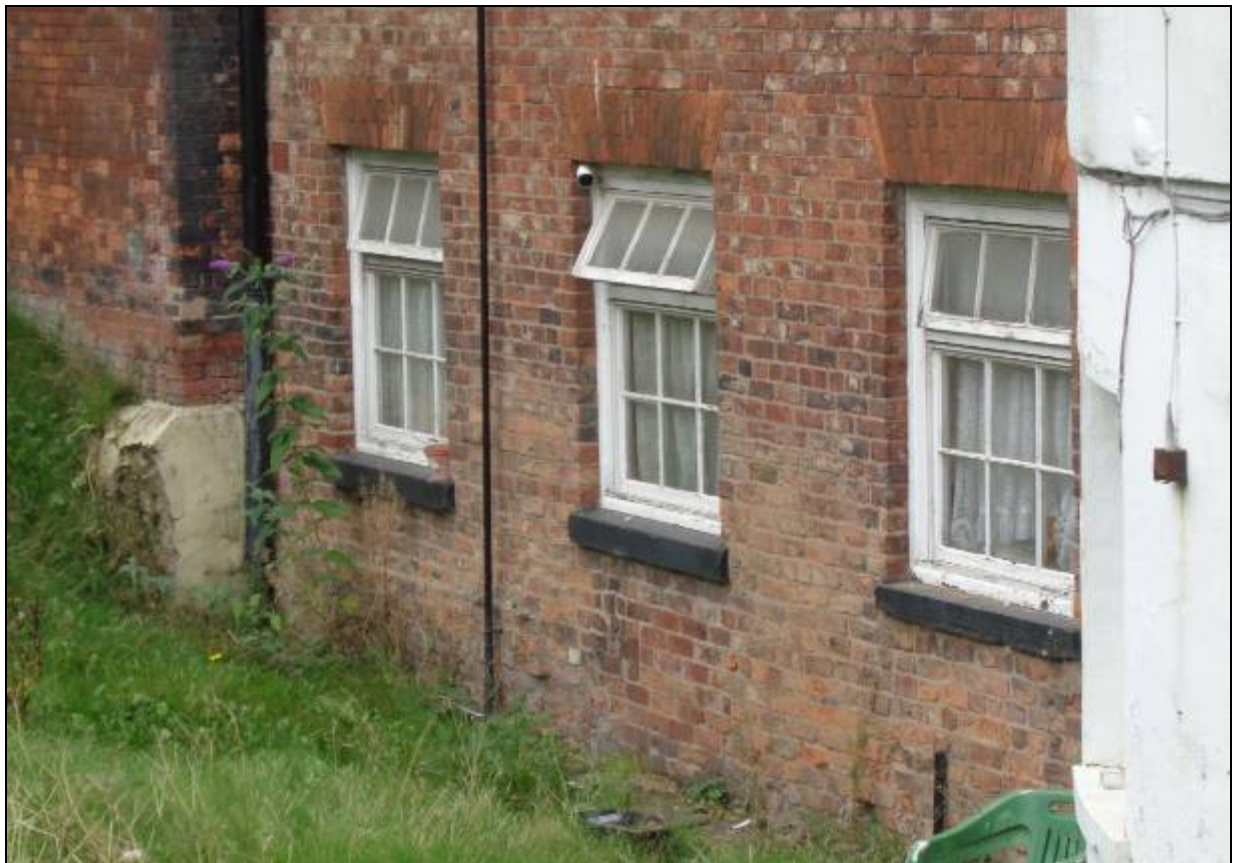
9. Late 20 th century casements in service wing basement are a notable exception
