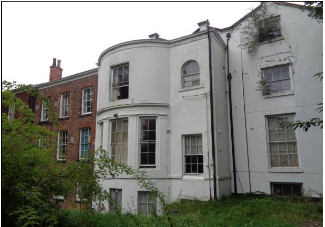
5. Rear of the main block with fine full-height bay window
