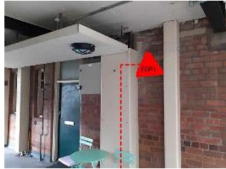
Picture showing cable route.
