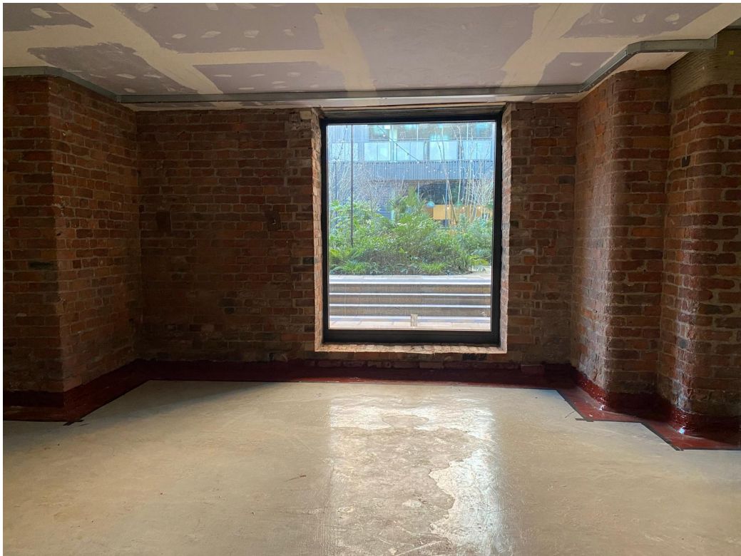
04 view of unit existing interior
