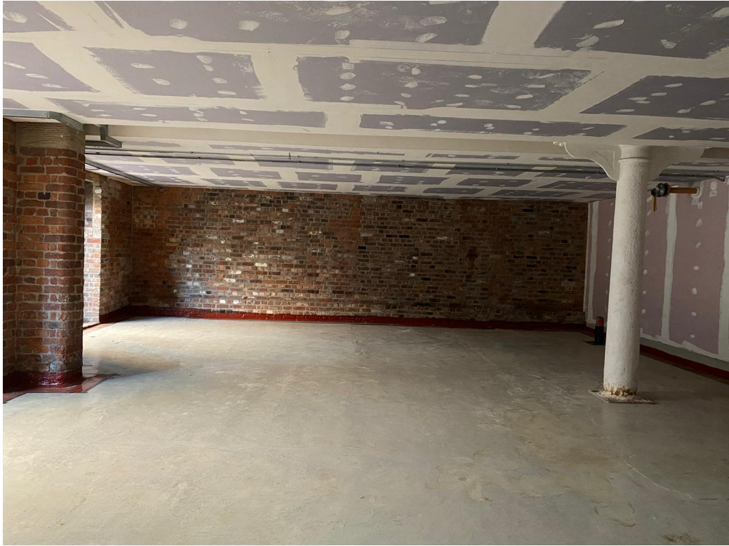
02 view of unit existing interior
