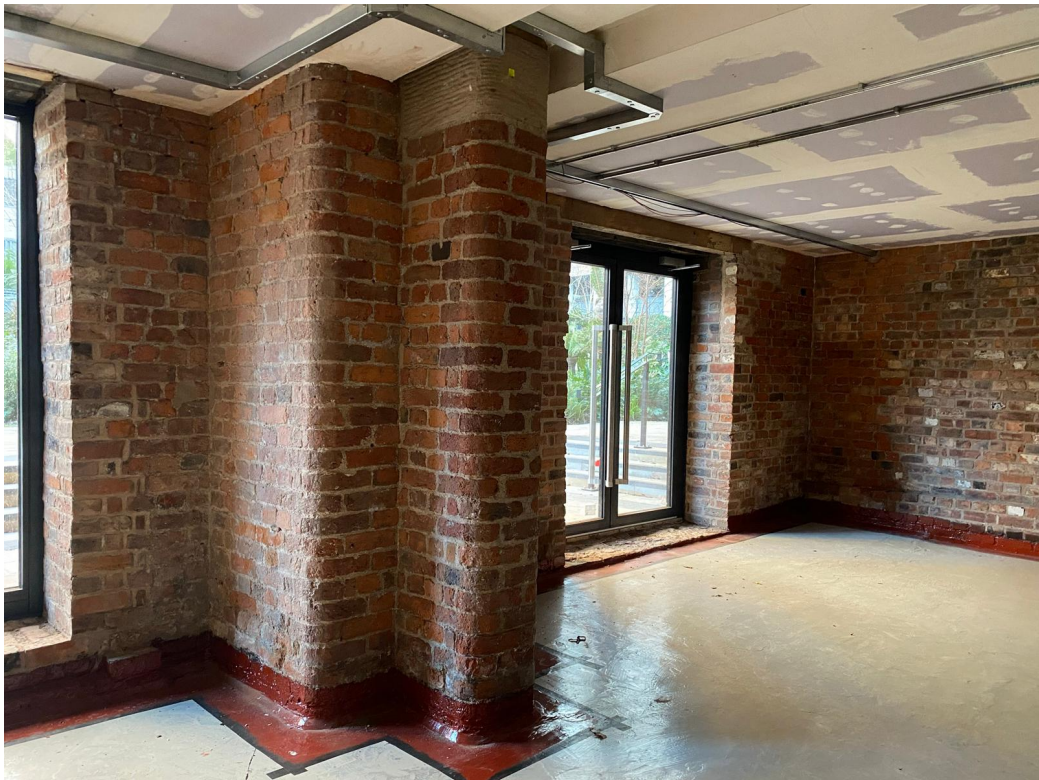
03 view of unit existing interior
