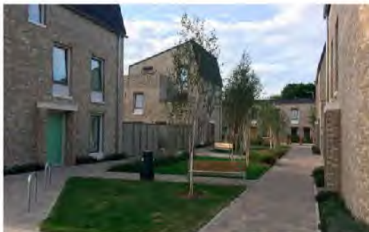
Safe, overlooked green spaces integrated into the development
