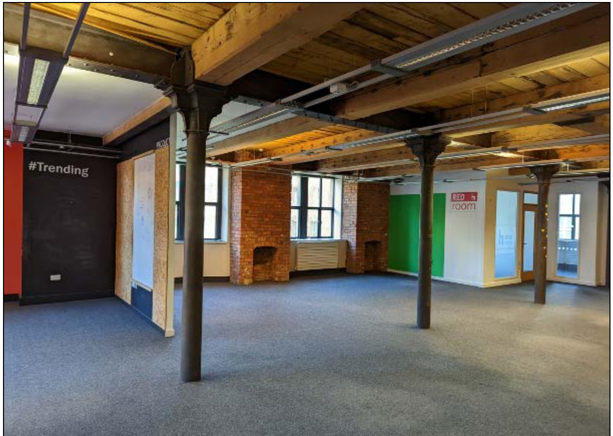
5. Third floor office space, showing original posts and beams
