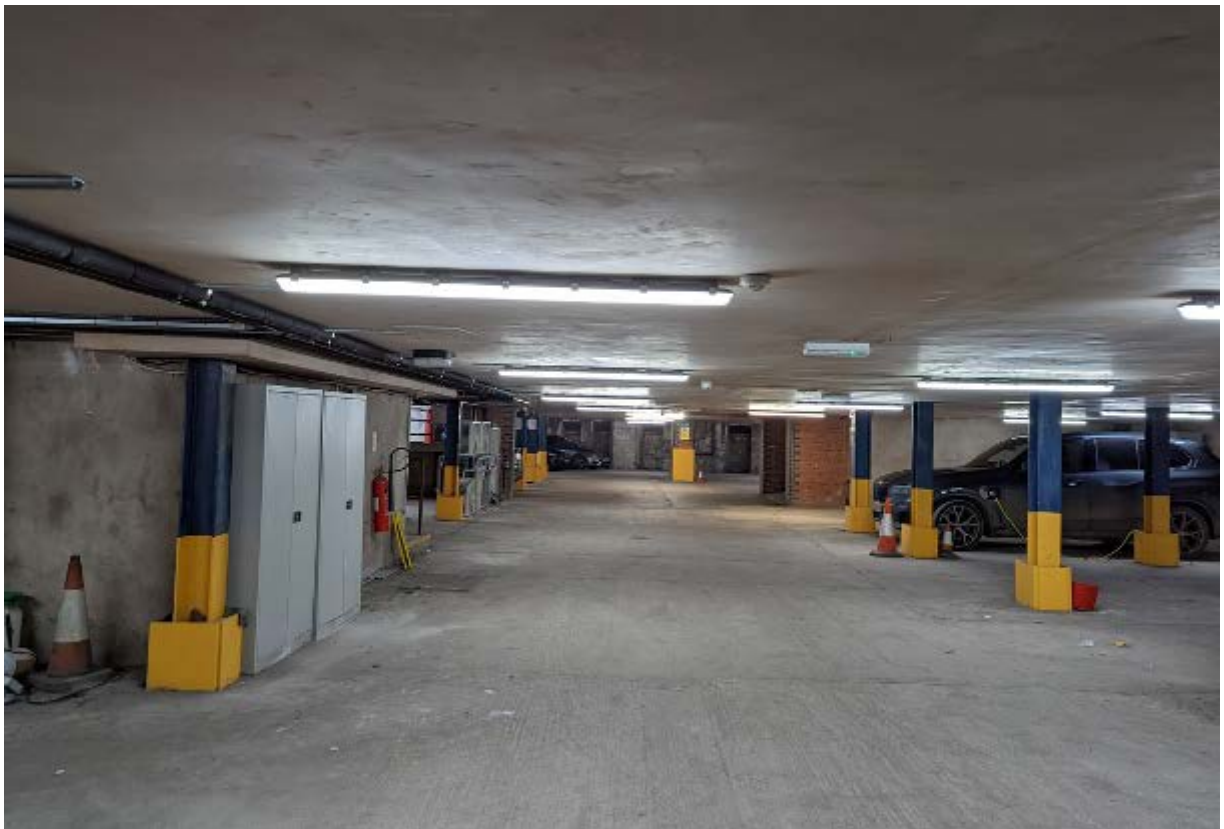
6. Basement is now used for car parking
