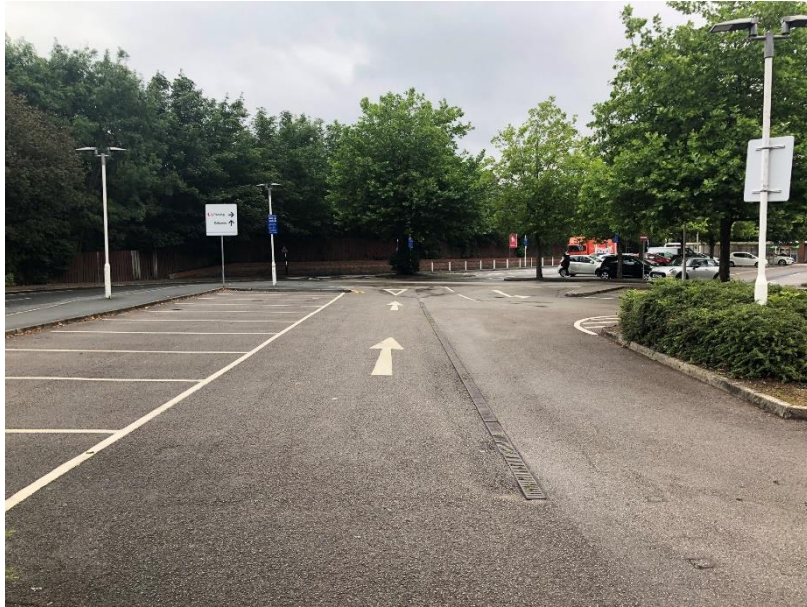
PLATE 1 SHOWING HARDSTANDING CARPARK
