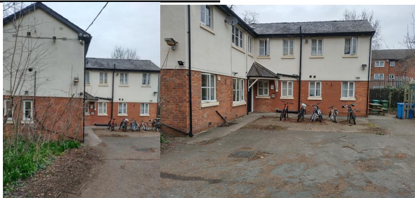
Fig. 1 – 76 Daisy Bank Road and 2 storey accommodation
